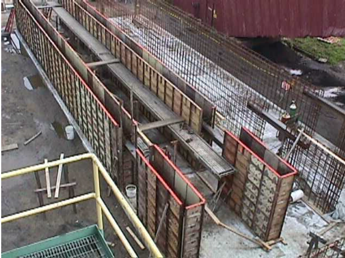
Figure 5. Forming the Walls of the Walking Floor Foundation
