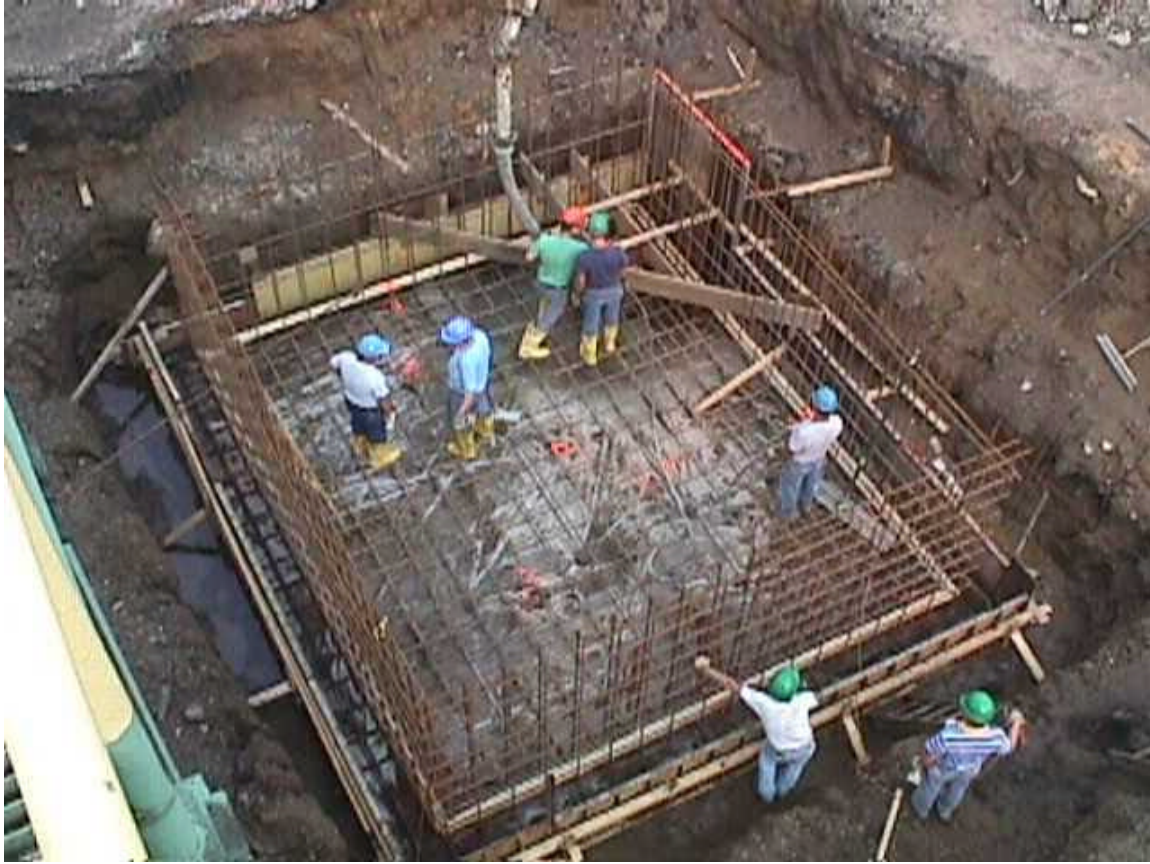
Figure 7. Installing Rebar in the Sawdust Receiving Pit, Under Construction
