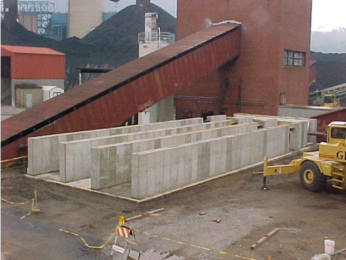
Figure 6. The Completed Walking Floor Foundation
