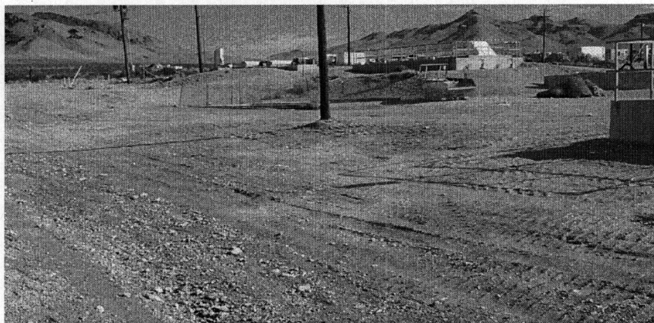
Upstream view on 27 Jan 2000, after backfilling.
