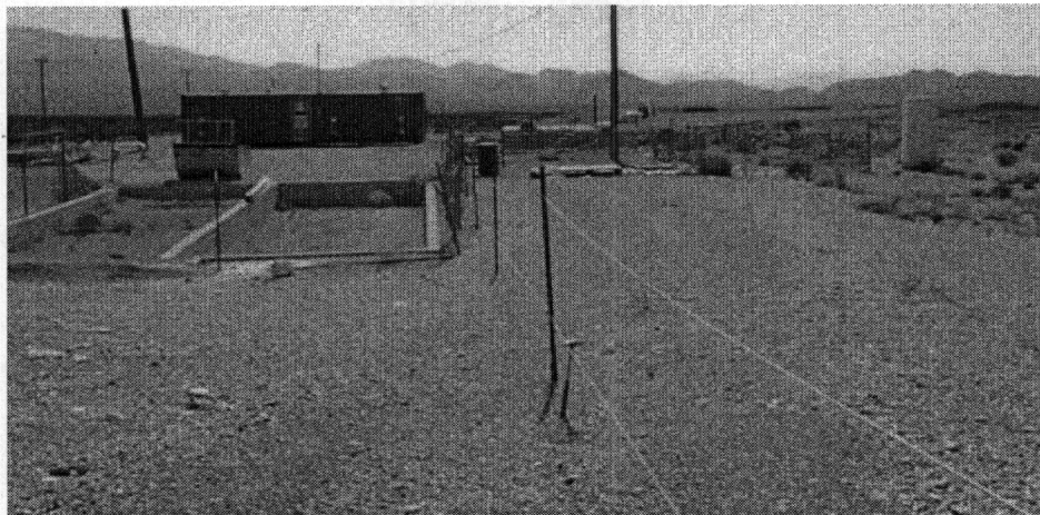
Downstream view on 06 Oct 1999, before excavation.
