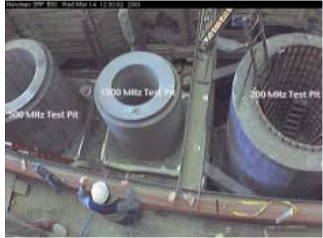
Figure 3: Test facility for 201.25-MHz SCRF cavities under construction at Cornell.
