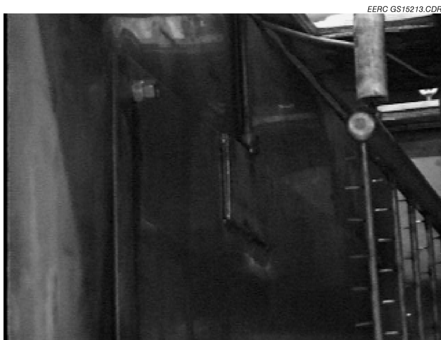
Figure 4.1-26. New rapper modification places the rapping force parallel to the surface of the ESP plate.
