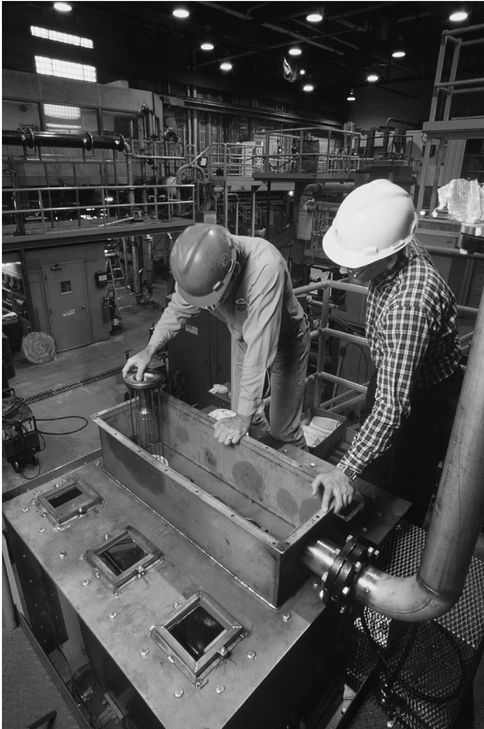
Figure 4.1-10. Outlet plenum during bag cage installation.
