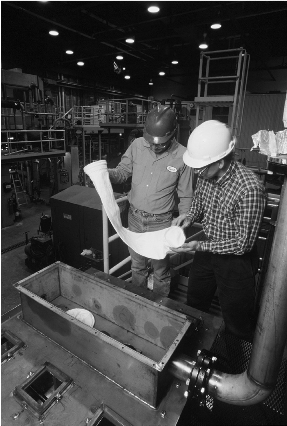
Figure 4.1-6. Outlet plenum during bag installation (notice the sight ports in the lower left of this picture).
