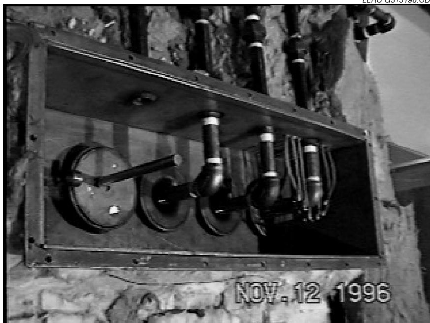
Figure 4.1-7. The pulse-jet bag-cleaning assembly modified to increase air volume released during a bag-cleaning cycle.
