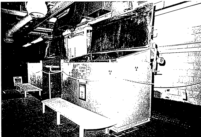
TANKS 9 AND 10--EFFLUENT COLLECTION TANKS
