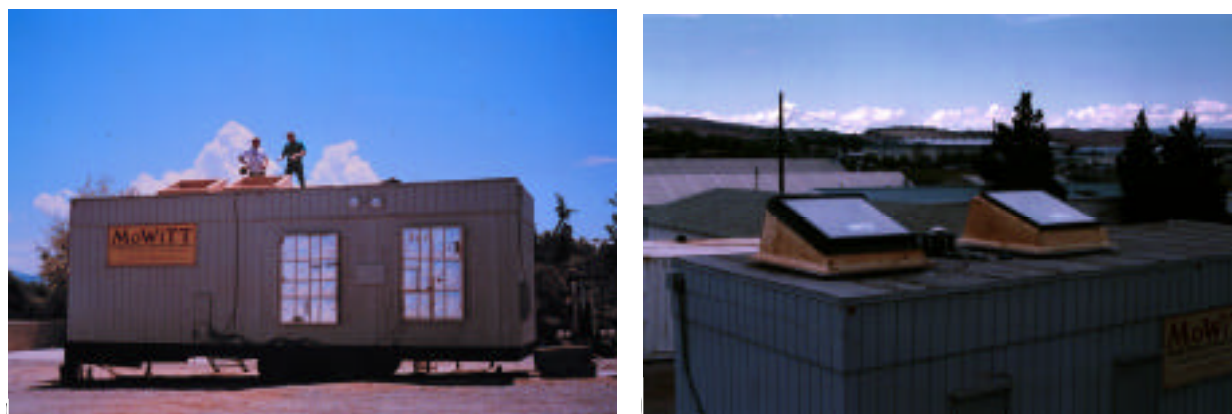
Figure 1. Conversion of the test facility to skylight operation. (a) Overall view from the north, before installation of the skylight adaptors. Here Chamber A is on the right. (b) View from the southwest during installation of the light wells on the chamber skylight ports. Chamber A is on the left.
