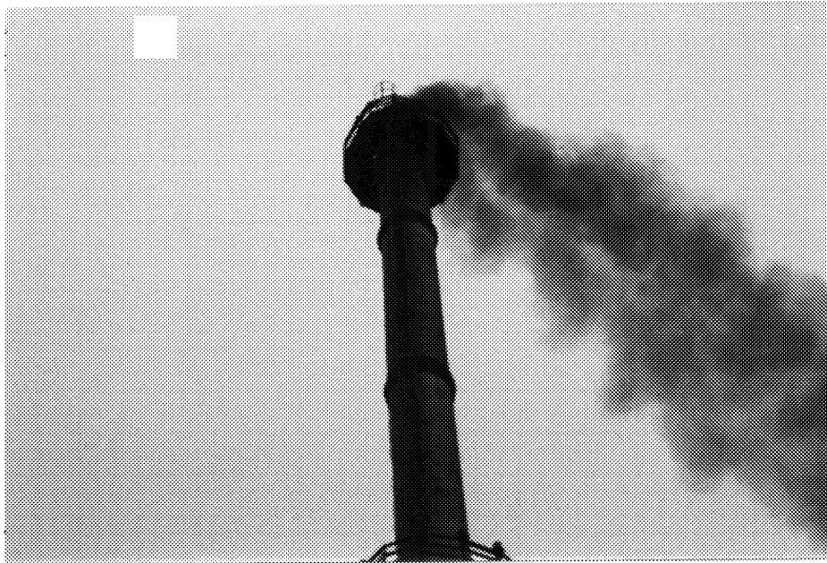
Figure 15. Stack Condition at Knurow Prior to Core Separator
