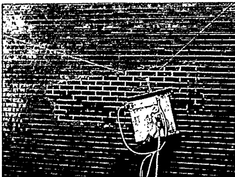
The Bartlett Robotic Climber removing the coating from a brick wall.
