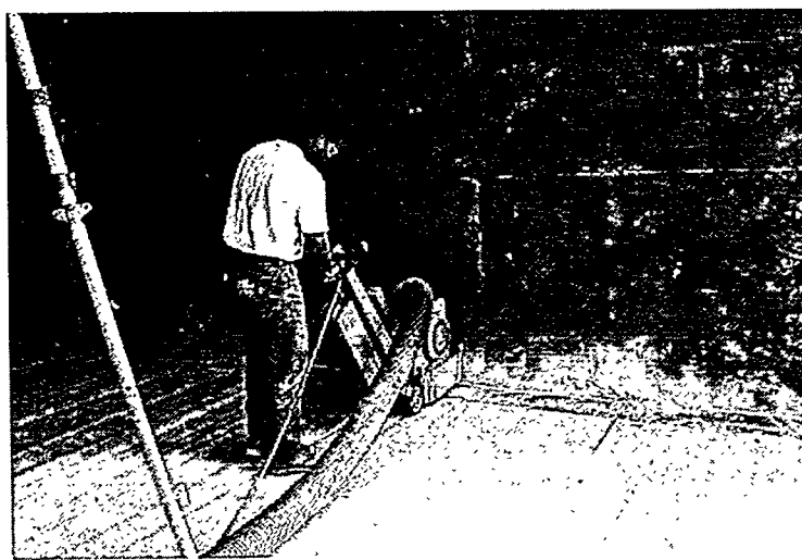
Figure 13. Marcris Floor Shaver operating on a coated concrete floor.
