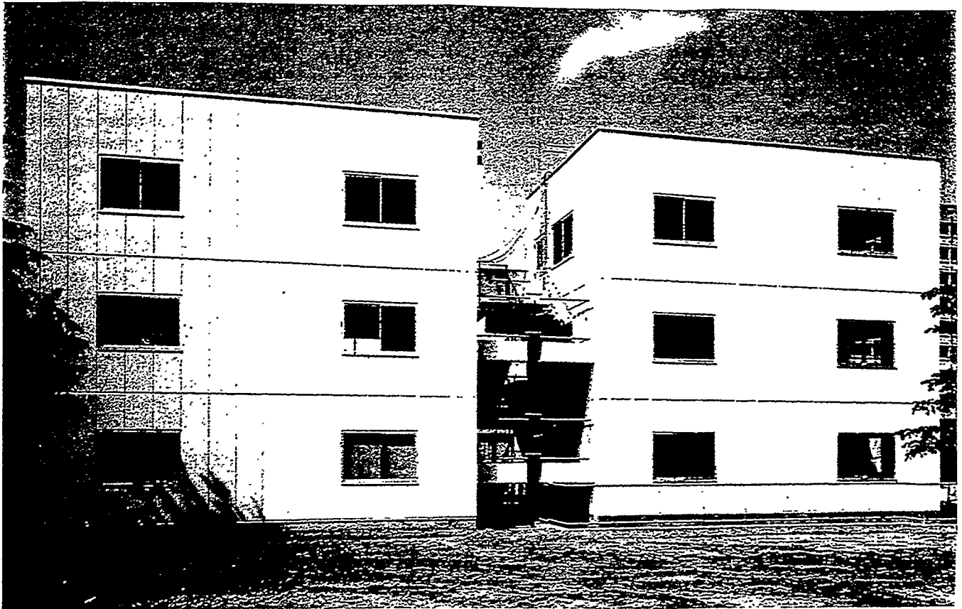
Full Scale Demonstration Buildings in Sendai, Japan Left: Fixed-Base Building Right: Base-Isolated Building
