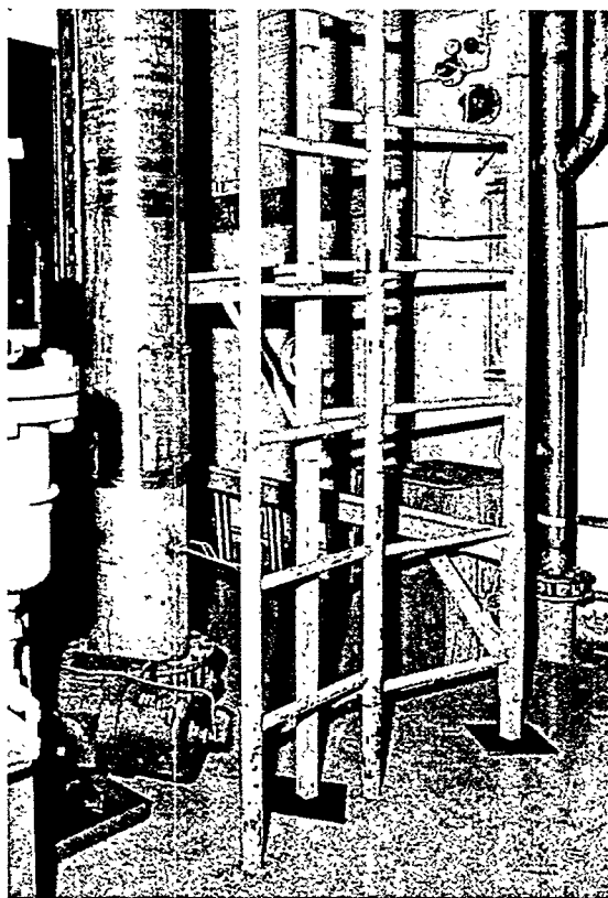
Figure 28. The vertical leg of the 250-mm-diameter building exhaust duct is shown to the left as it enters the floor of the Assembly Room. Just below grade, the line curves and leads horizontally under the wall seen to the right background. The cover plate (seen on the right side of the duct in the middle of the photograph) was later installed over the hole cut into this line to view for the first time the extent of this contamination incident. Close inspection above that patch shows the weld seam when the length of exhaust line was reinstalled after completing cleanout. The horizontal object at the bottom where the duct enters the floor is the butterfly valve discussed to in the text.
