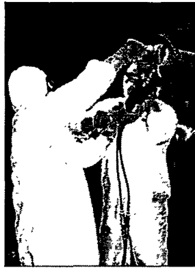
Figure 4 LANL Technicians Cut Pipe Legs from Glovebox Mockup
