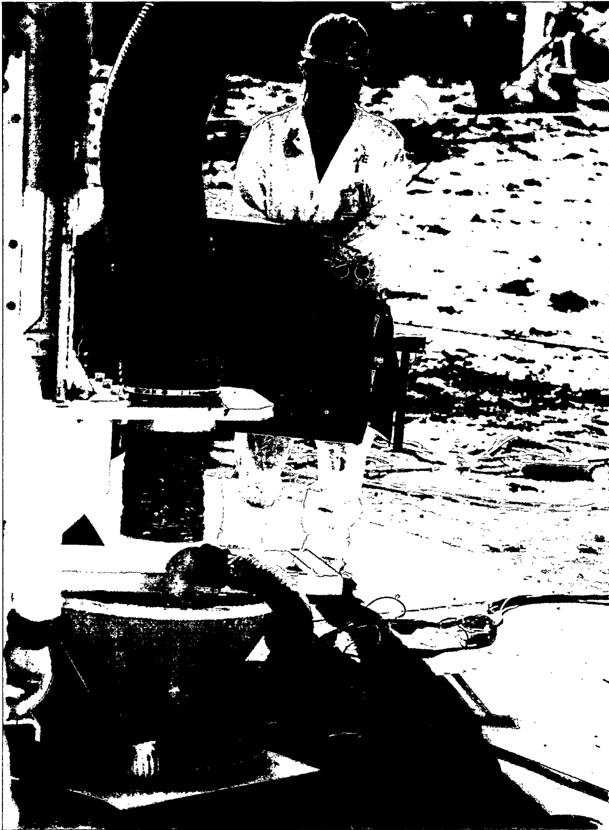
Figure 16. Worker monitors the grouting operation (Photo 97-789-1-23).
