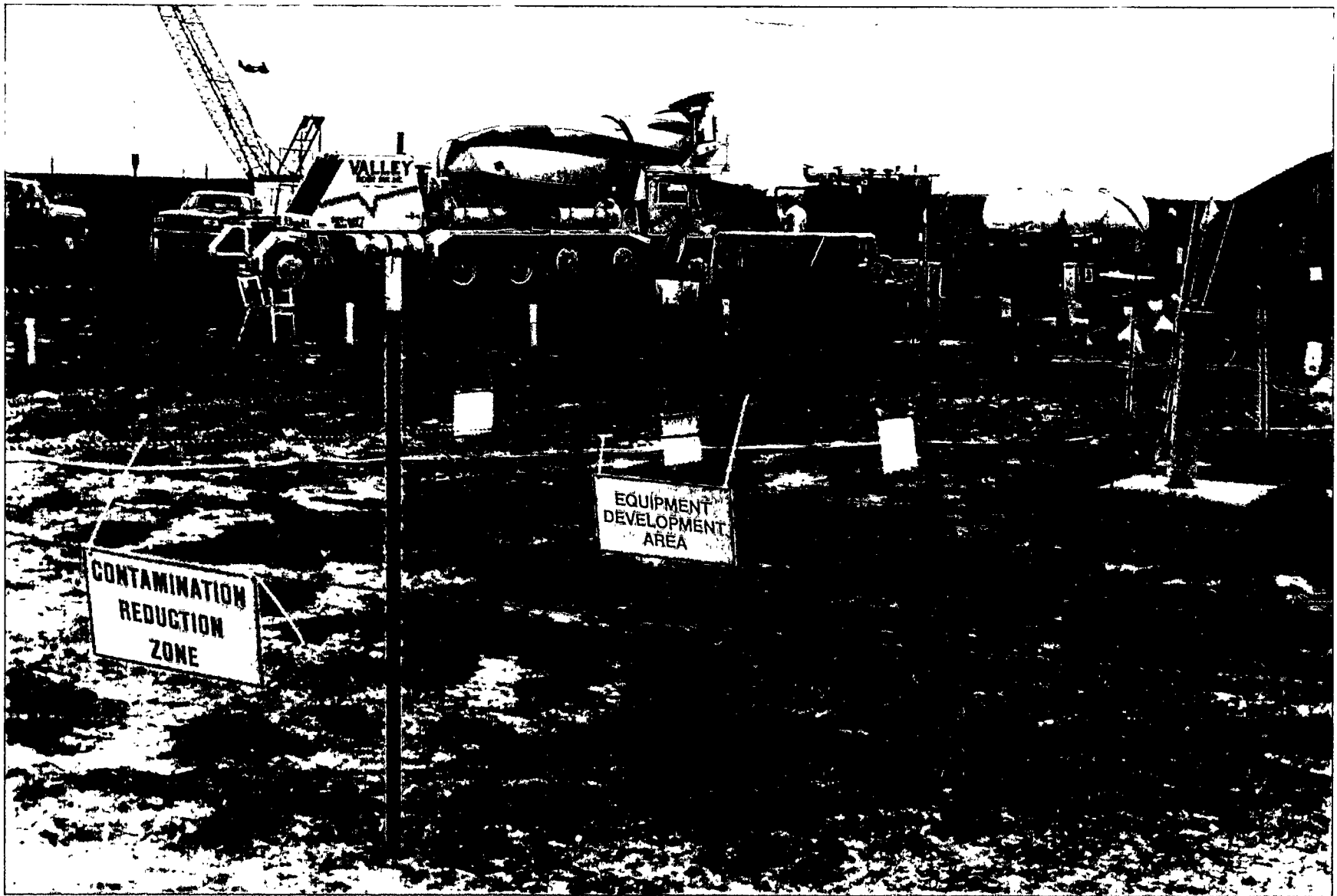
Figure 11. Exclusion zones established for Acid Pit stabilization showing cement truck and pumps outside the zones (Photo 97-791-1-8).
