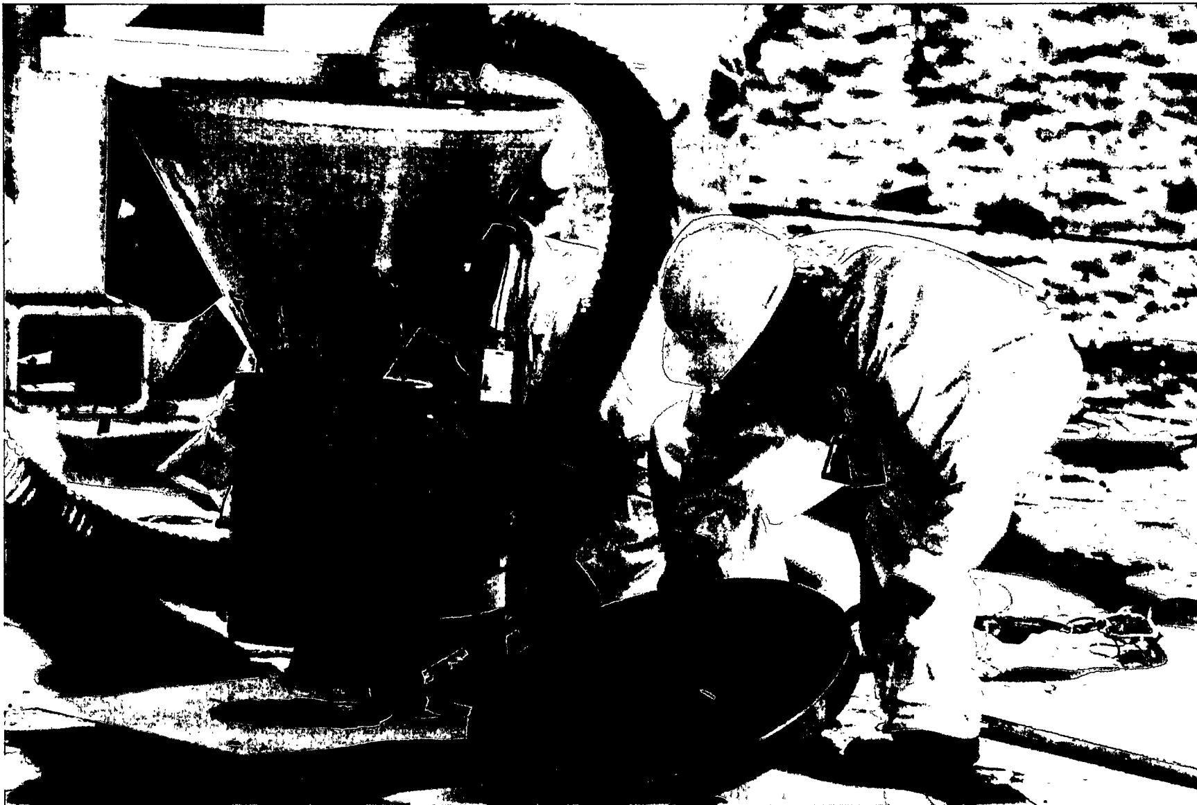
Figure 18. Placing the catch pan and blotter paper over a new hole and cleaning the old hole (Photo 97-789-1-11).
