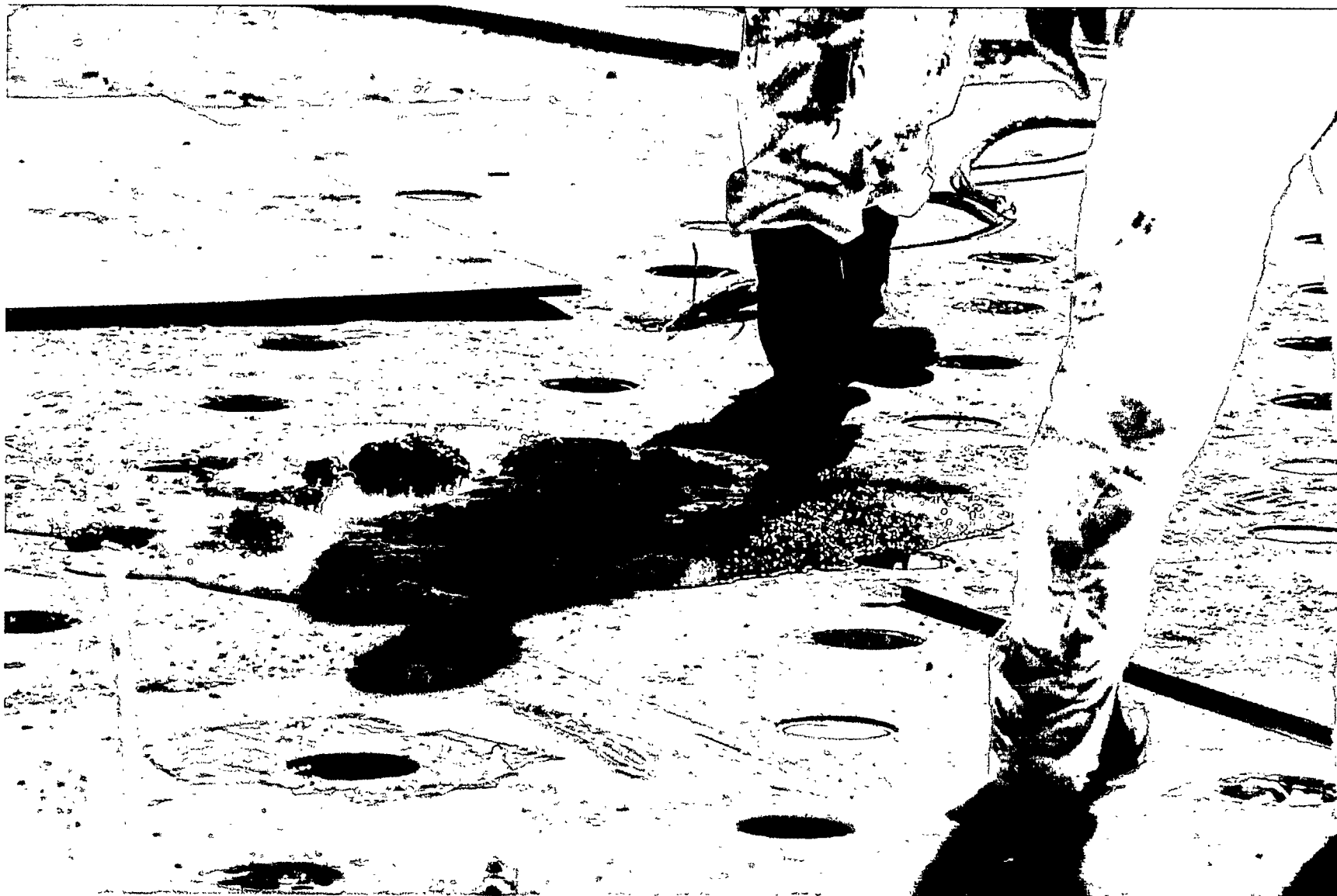
Figure 33. Grout returns during Acid Pit grouting (Photo 97-789-2-12).
