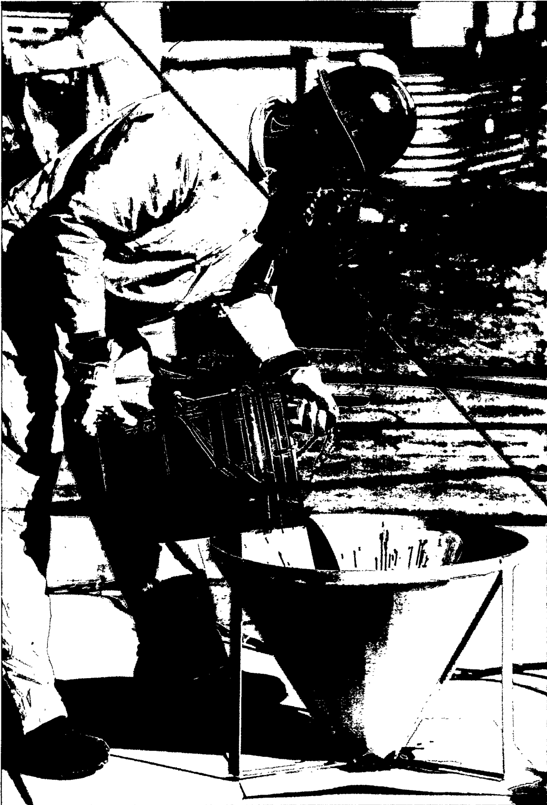
Figure 14. Worker pouring catch cup material into an unused hole in the thrust block (Photo 97-789-2-8).
