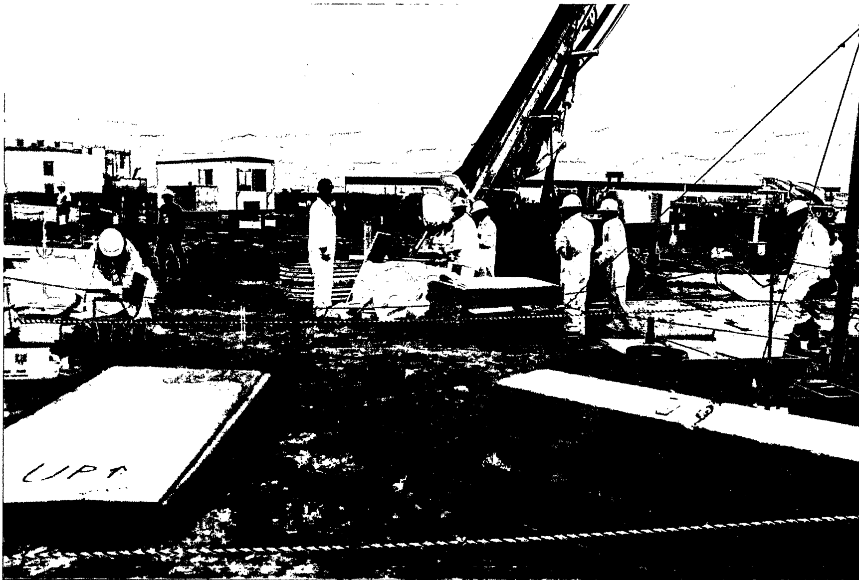
Figure 19. Positioning the drill stem over the cleanout trough (Photo 97-791-1-23).
