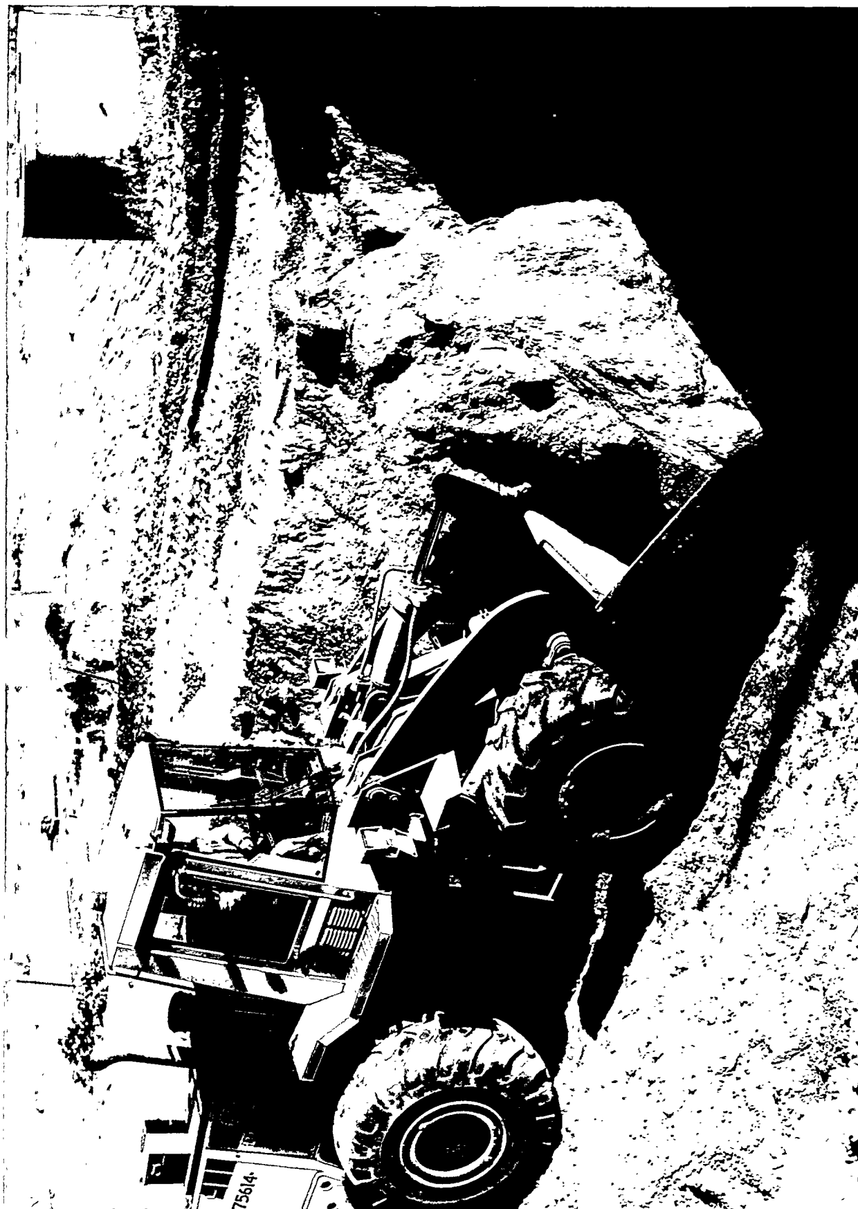
Figure 29. Operational Readiness Pit monolith being excavated intact (Photo 97-835-1-25).
