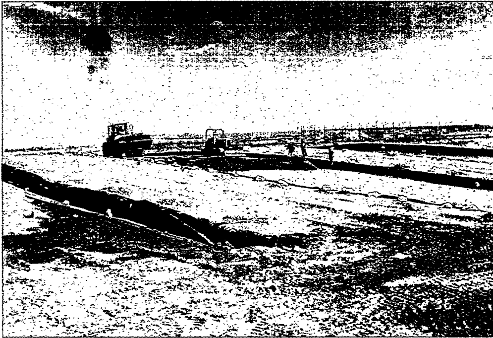
Figure 13. Capillary Barrier Installation
