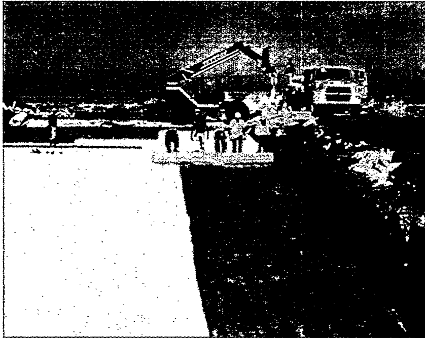
Figure 10. GCL Installation
