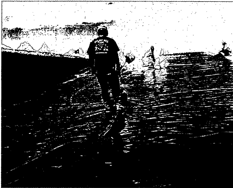
Figure 8. Welding Seams of Geomembrane Panels
