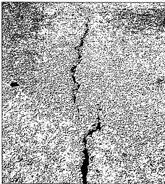
Figure 6. Longitudinal Cracking due to Differential Settlement
