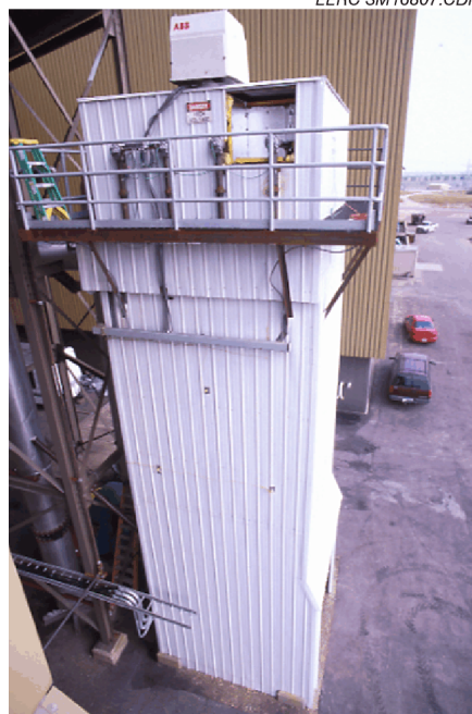
Figure 5. AHPC showing access platform and HV power supply.
