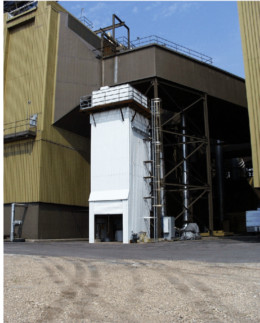
Figure 4. AHPC installed at the ESP inlet at the Big Stone plant.
