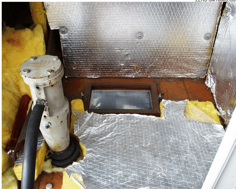
Figure 7. Pneumatic plate rapper and sight port at top of AHPC.
