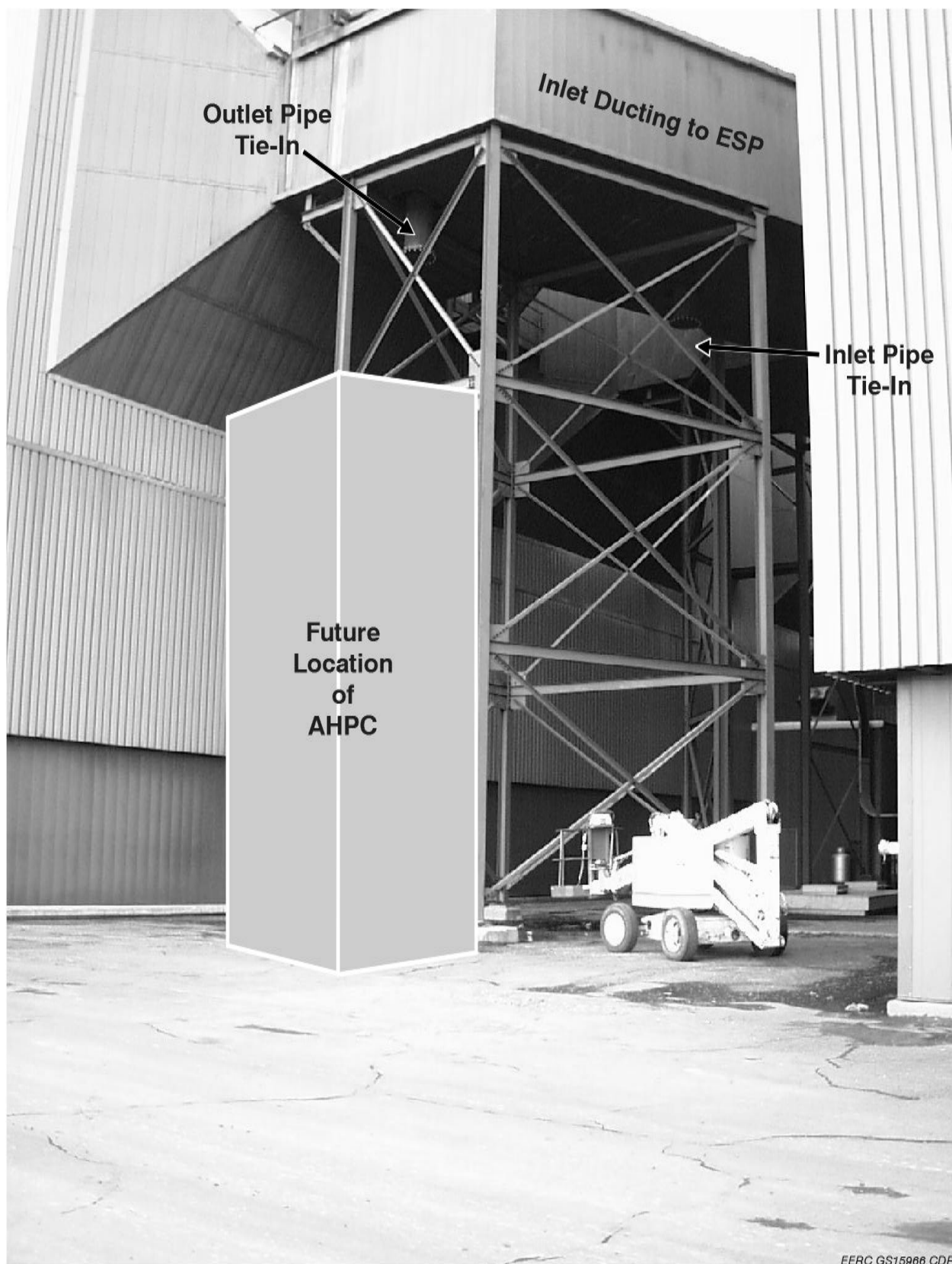
Figure 1. Inlet and outlet ports from the underside of the main ESP inlet duct.
