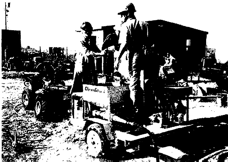
Figure 14. Mixing grout at Sandia.
