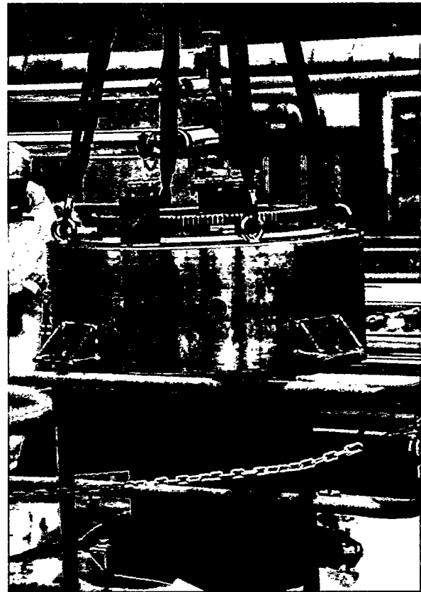
Fig. 7-2. Installing the charge vessel into the west manhole extension of Tank C-2.
