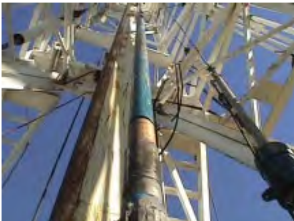
Fig. 15. DOE Motor In Derrick
