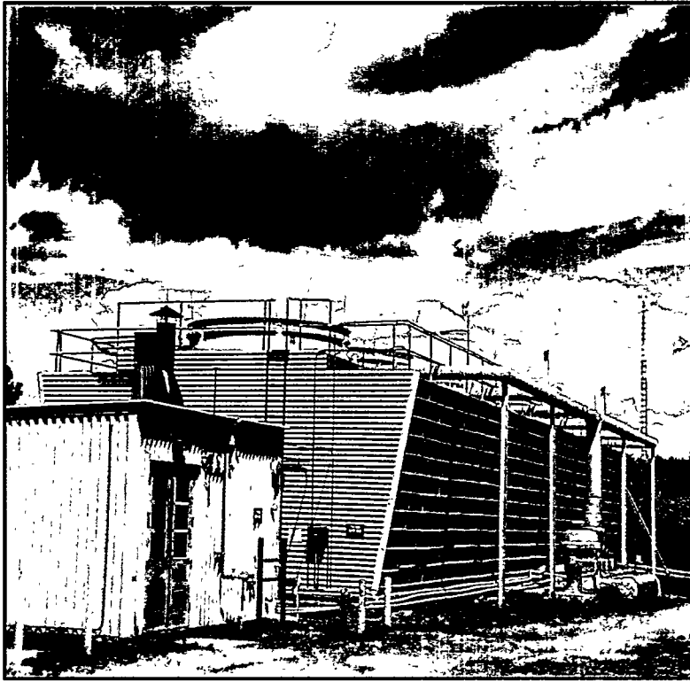
Fig. 7-3. Cooling tower at TA-53.
