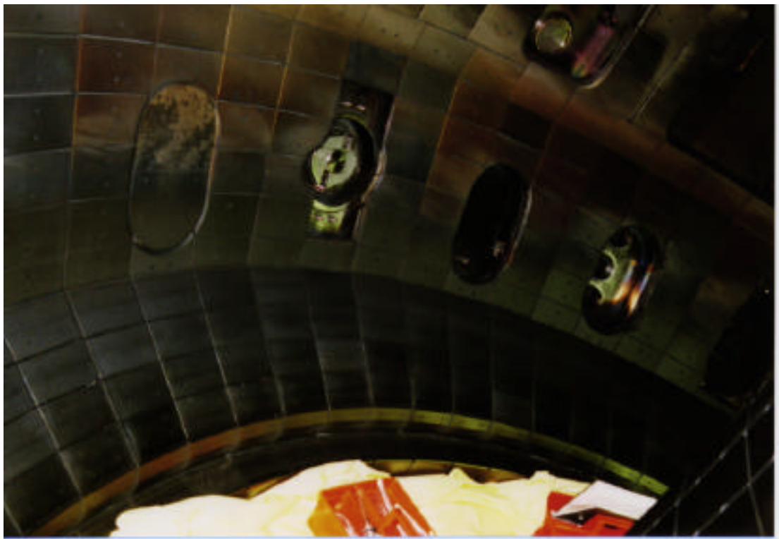
Figure 2.11. Photograph of the 0 – 90° R-1 access ports.
