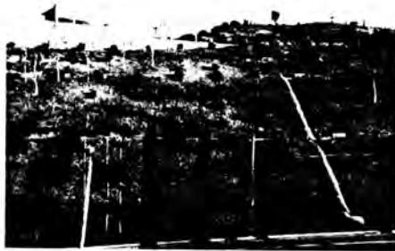
FIG. 2. Conventionally Graded Hill Slope with Planar Face, Rectilinear Drainage Ditch, and uniformly Spaced Plantings
