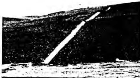
FIG. 1. Conventional Grading with Planar Slopes and Rectilinear Drainage Ditch in Highly Visible and Exposed Location
