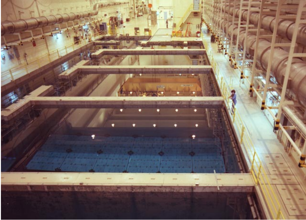
FIGURE 5. The INEEL is a key DOE resource for managing spent nuclear fuel. This underwater fuel storage facility at INEEL receives and stores DOE-owned spent nuclear fuel from several sources, including the U.S. Navy and the INEEL's Advanced Test Reactor.
