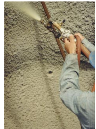
FIGURE 18. INEEL researchers find science-based solutions to DOE's environmental cleanup challenges. Here, naturally occurring microbes are used to clean radioactively contaminated walls and ceilings at a reactor in the United Kingdom.
