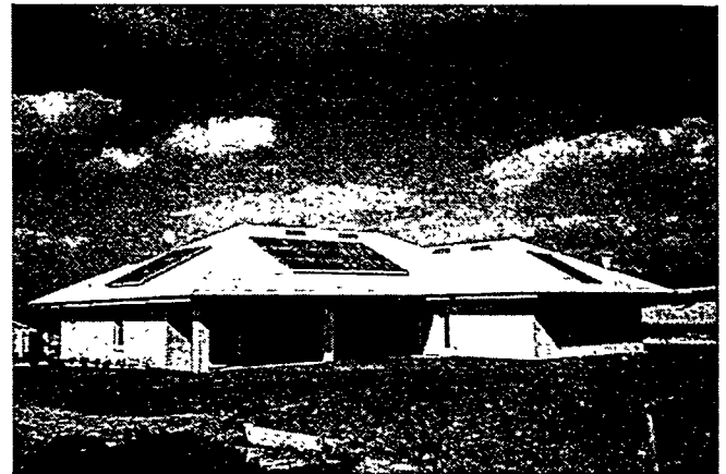
Figure 5. A super-energy efficient, utility-interactive photovoltaic residence in Lakeland, Florida.
