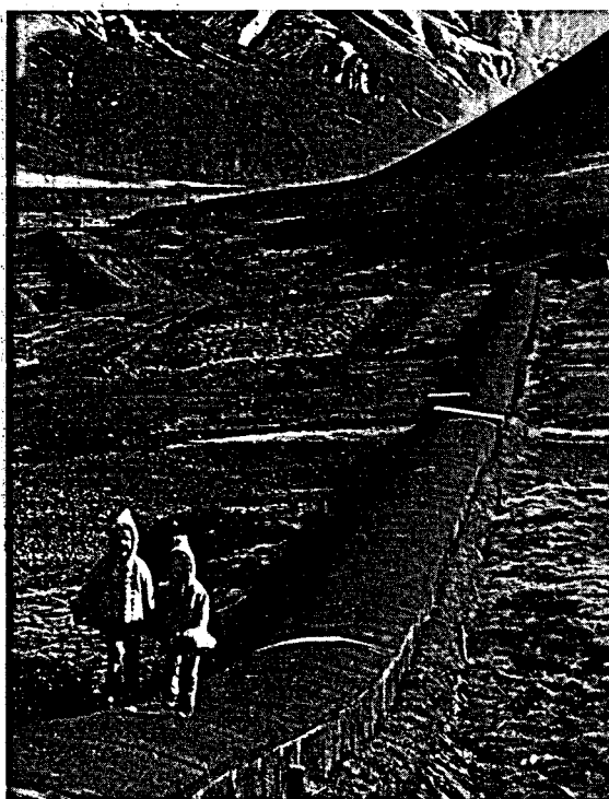
Figure 13. Pipeline conduit from Reykir to Reykjavik, 10 miles of 2" X 14" pipe.
