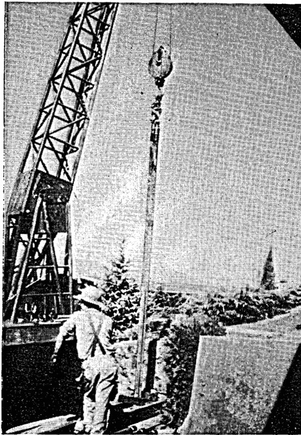
PHOTOGRAPH 7. Pulling Heating Pipes for Repair
