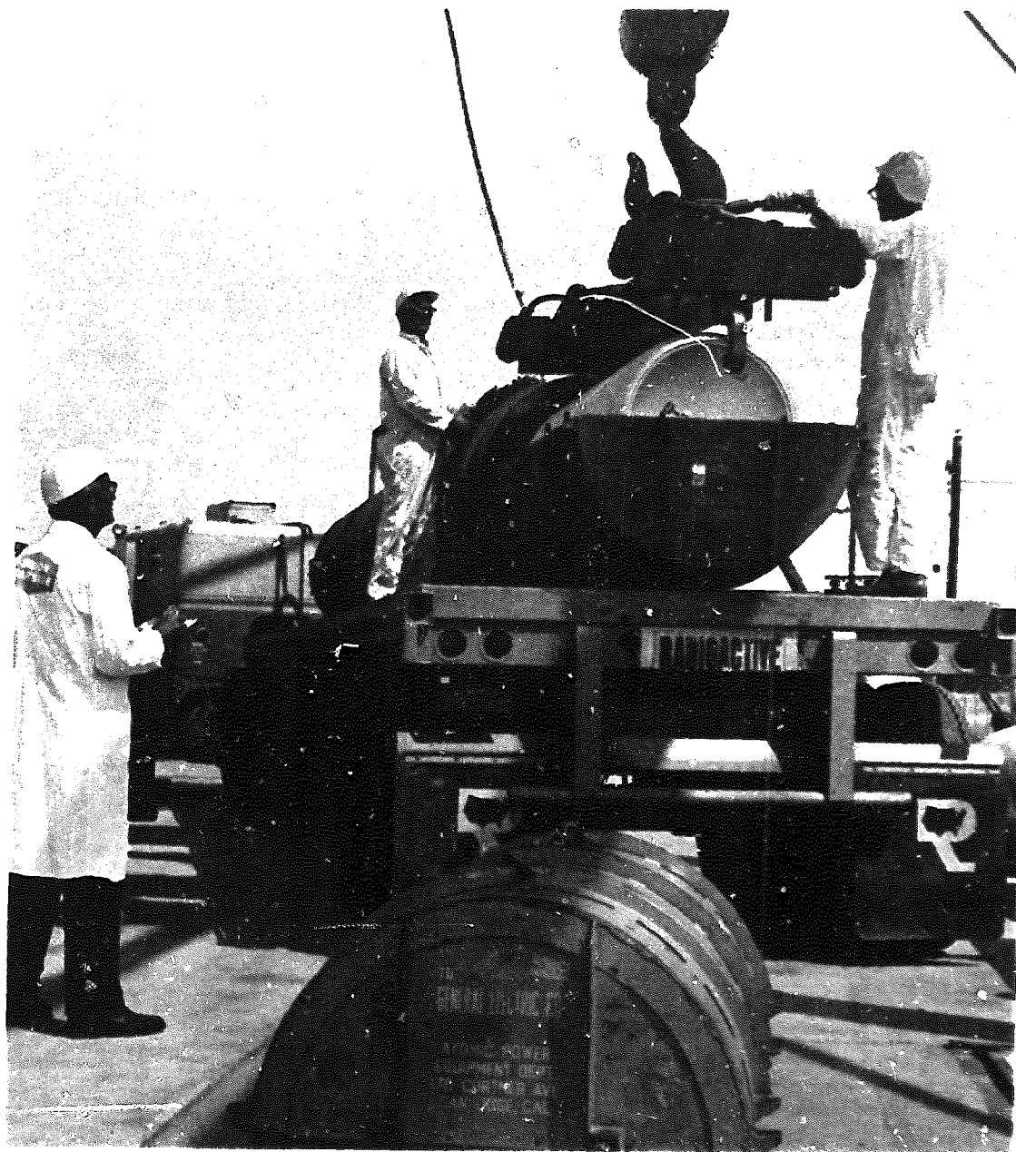
Figure 10 Typical \text{UF}_6 Shipping Container and Protective Carrier for Enriched Uranium. (Capacity: 2½ tons of \approx 5% Enriched \text{UF}_6 .)
