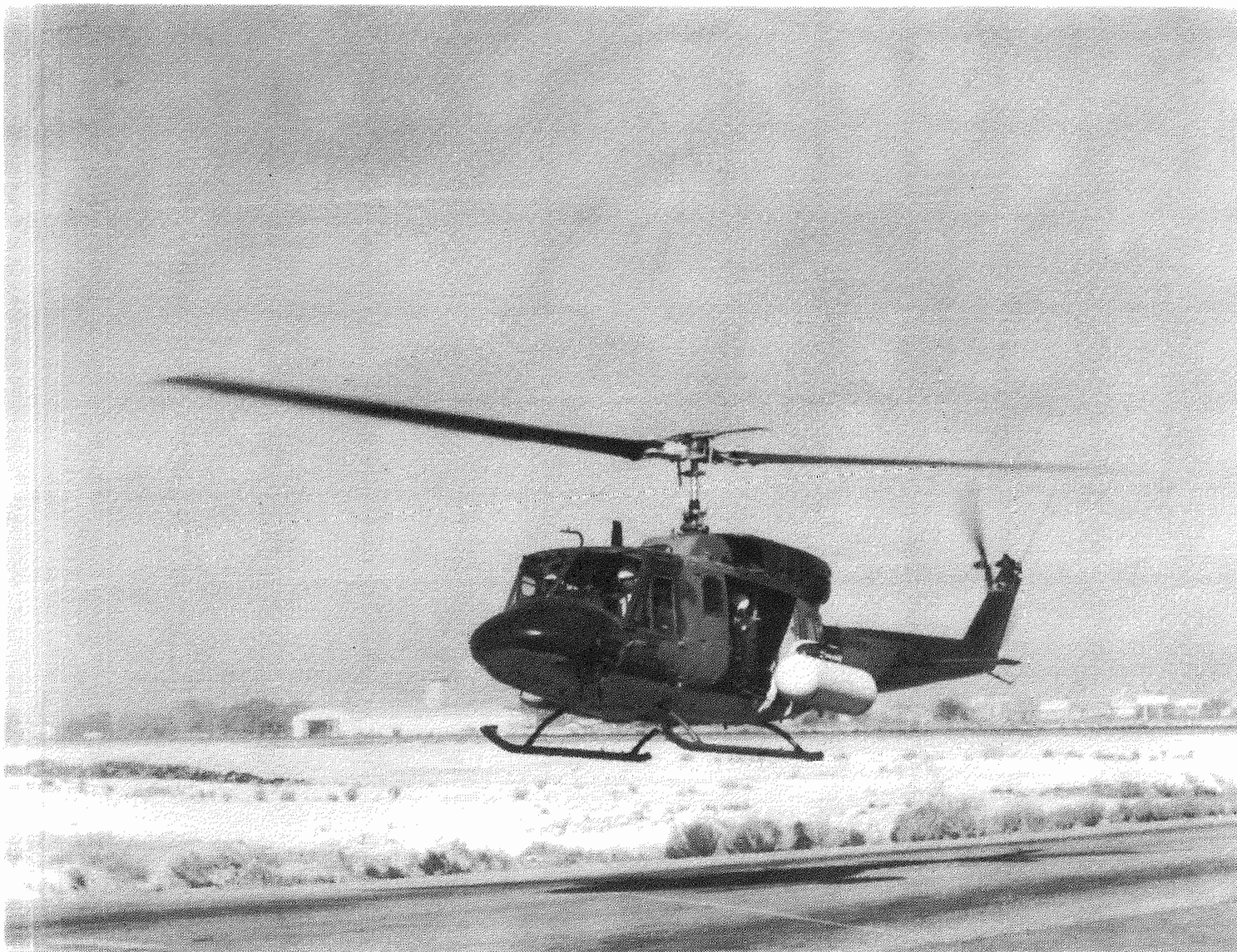
Figure 3. The Air Force HU-1N equipped with two gamma detector pods.
