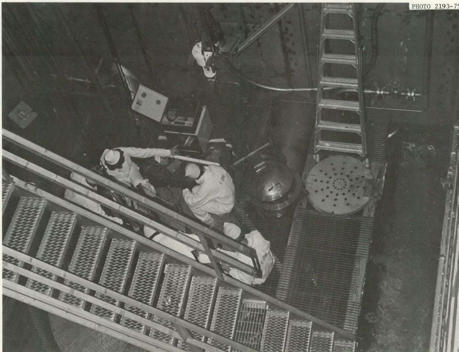
Figure 46. Inspection Engineering Personnel Videotaping Underwater Reactor Components
