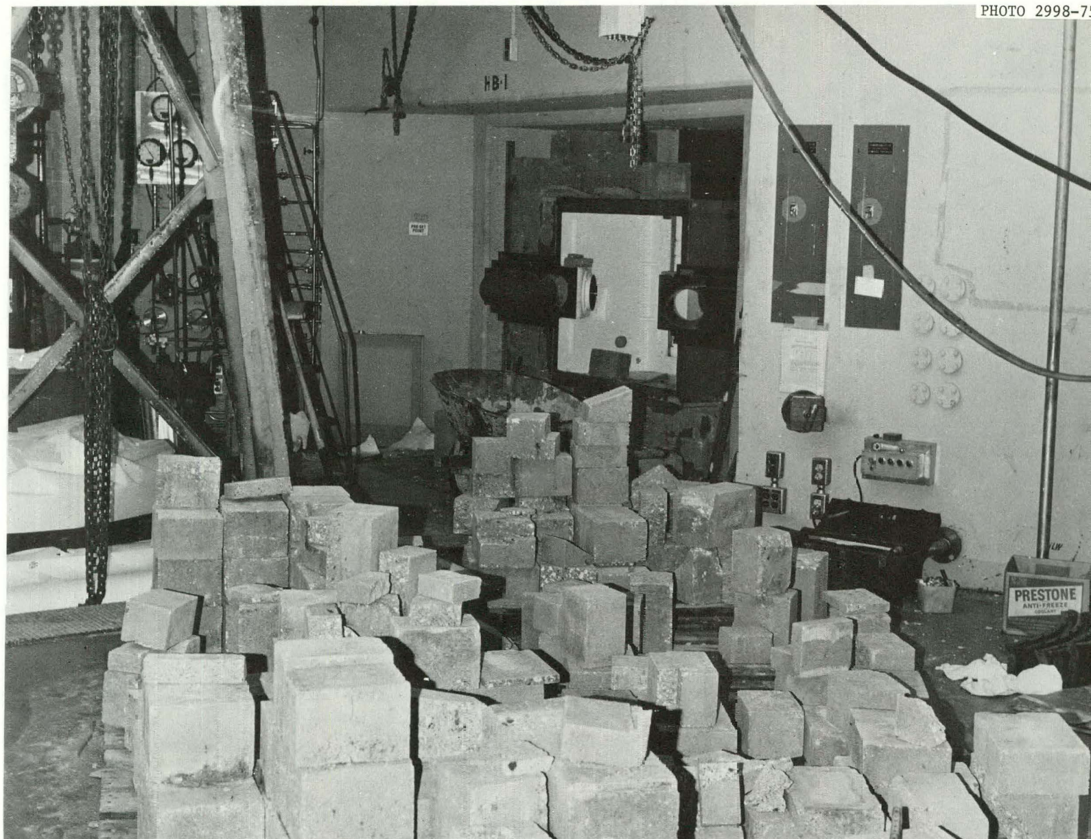
Figure 61. Shielding Blocks for Beam Tube Facility
