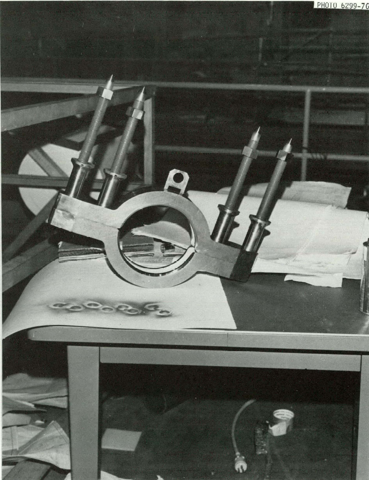
Figure 53. One of Two Four-Bolt Marman Clamps Used on the EF-2 Facility
