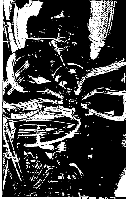
◀◀ These low-NO x burners, installed at the Cherokee Station, are capable of firing gas or coal. Long-term tests conducted throughout 1994 showed that combined GR-LNB achieved NO x reductions of 60–73%. The natural gas supply lines meet the flue gas recirculating line at the points of intersection just outside of the boiler wall.
