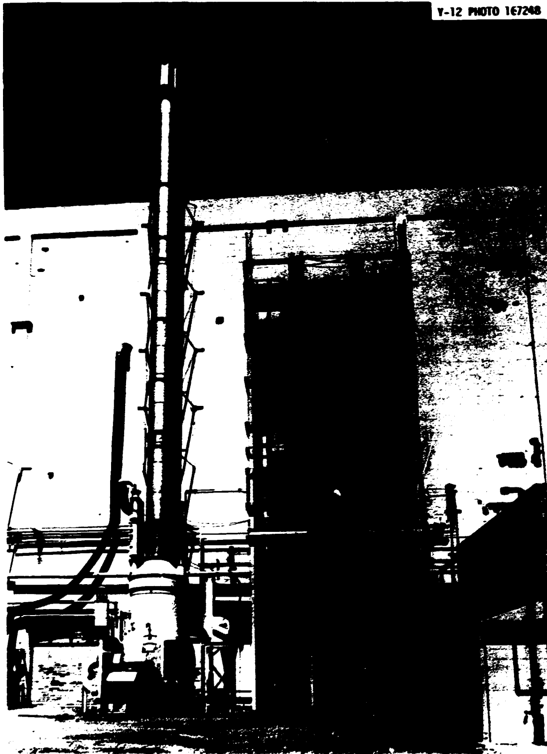
Fig. 5.4. Potassium boiler module installed in equipment tower.
