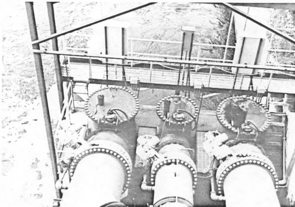
Figure F-4 Pocono Lake - Inlet Valves and Turbine Casings
