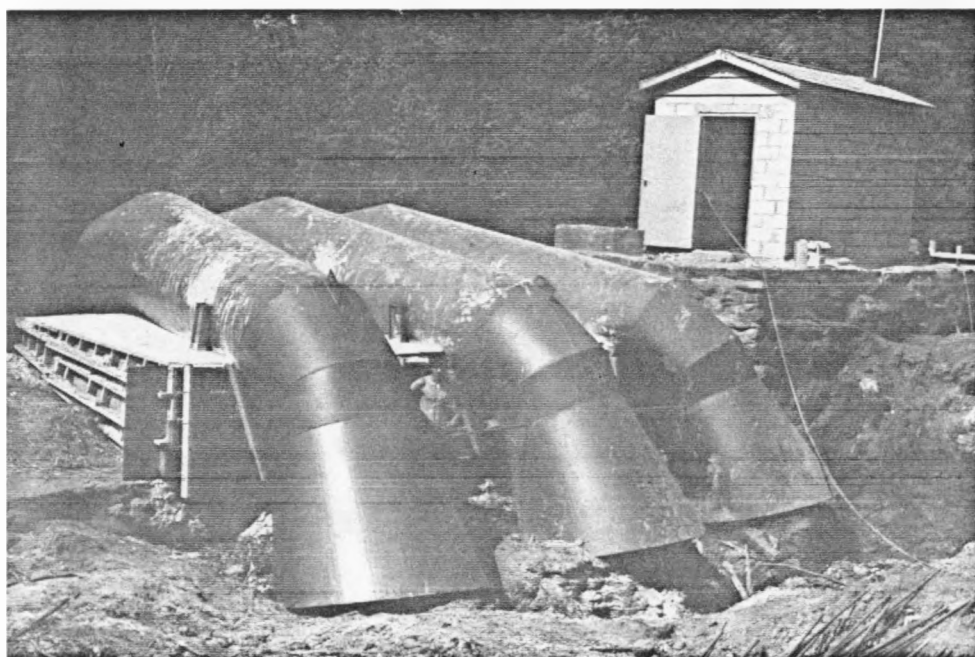
Figure 5-3 Placing of Concrete Support for Penstocks at Second Broad River Hydroelectric Project
