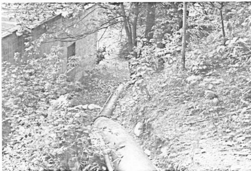
Figure J-2 Tierckenkill Falls - Penstock Between Dam and Powerhouse
