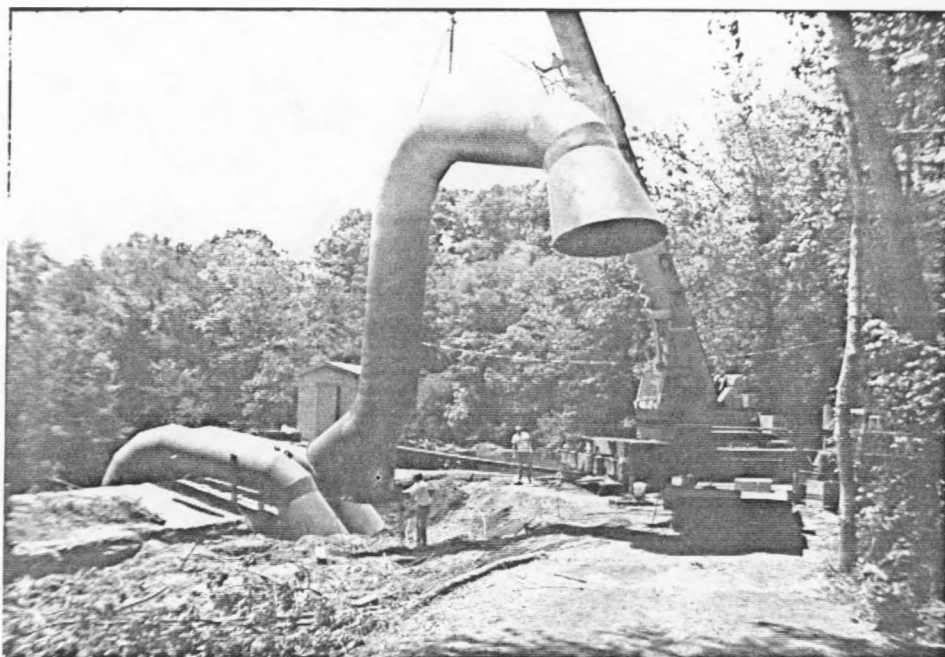
Figure 5-2 Installation of Siphon Penstocks at Second Broad River Hydroelectric Project
