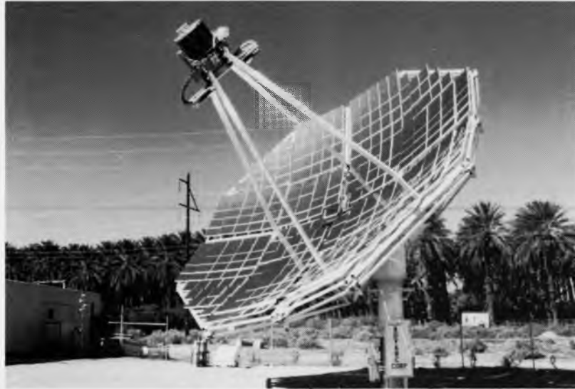
Figure 1. Advanco-Vanguard dish-Stirling module in operation. This module currently holds the world record for sunlight-to-grid-power conversion efficiency at 29.4%.
