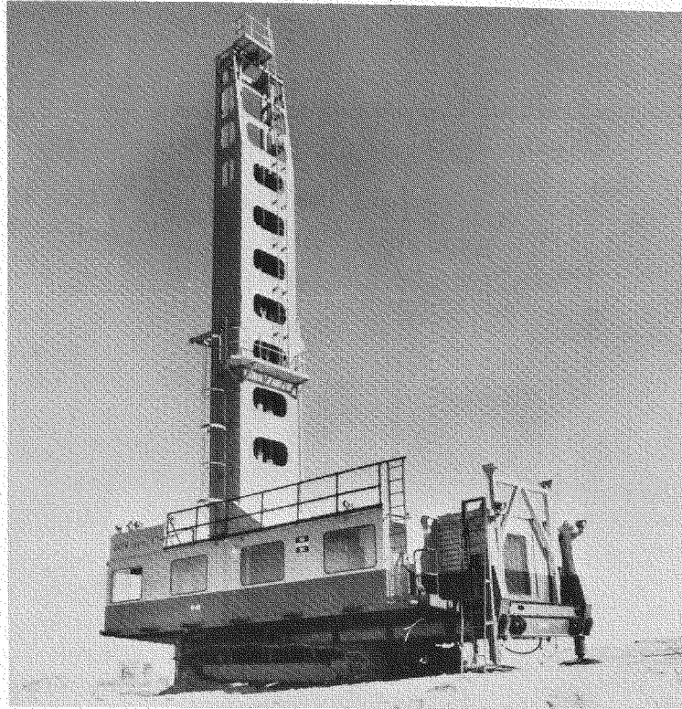
Figure 7. Rotary Drill for Overburden Drilling
