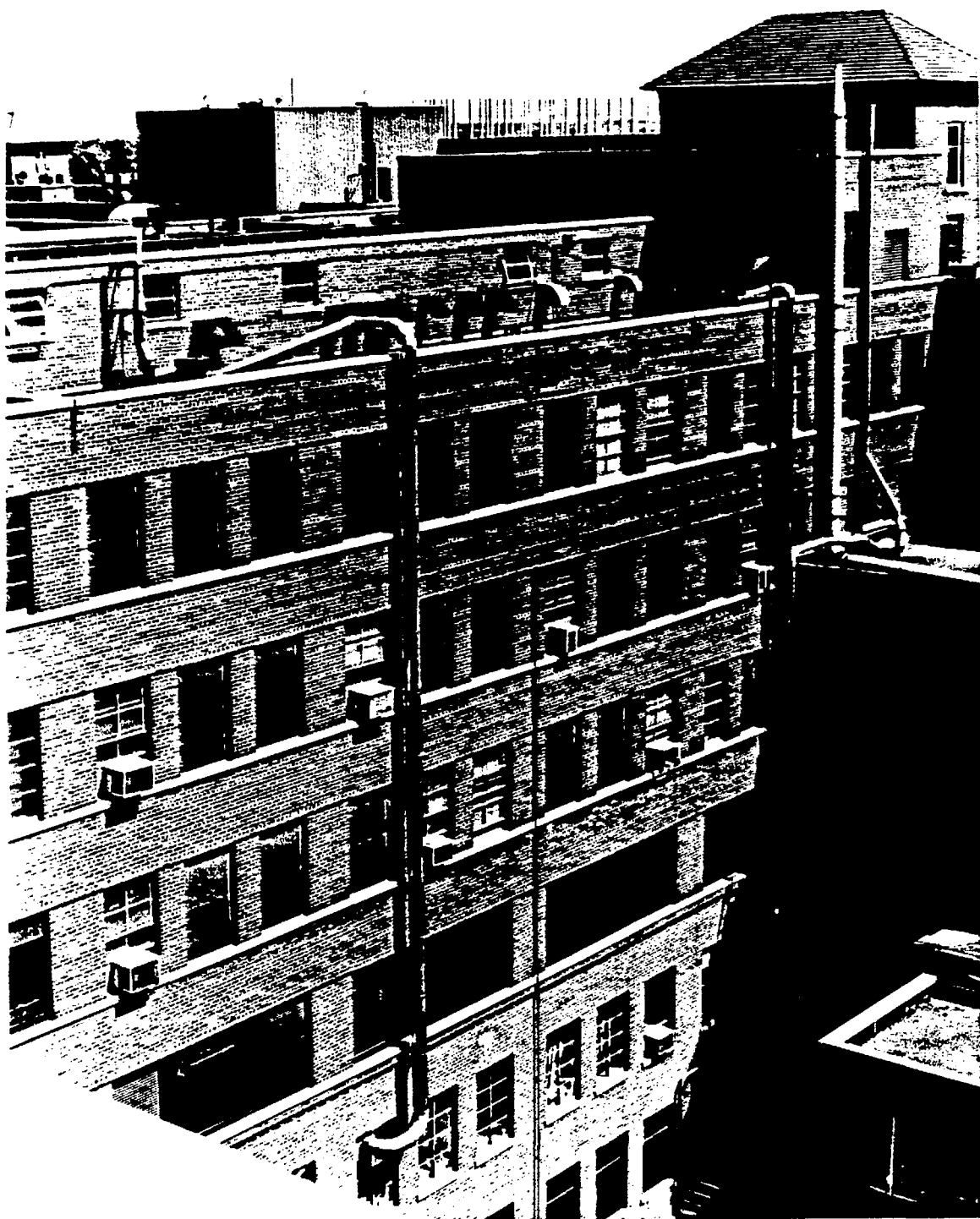
Figure 4 Effluent Release Points on Bldg. 55
