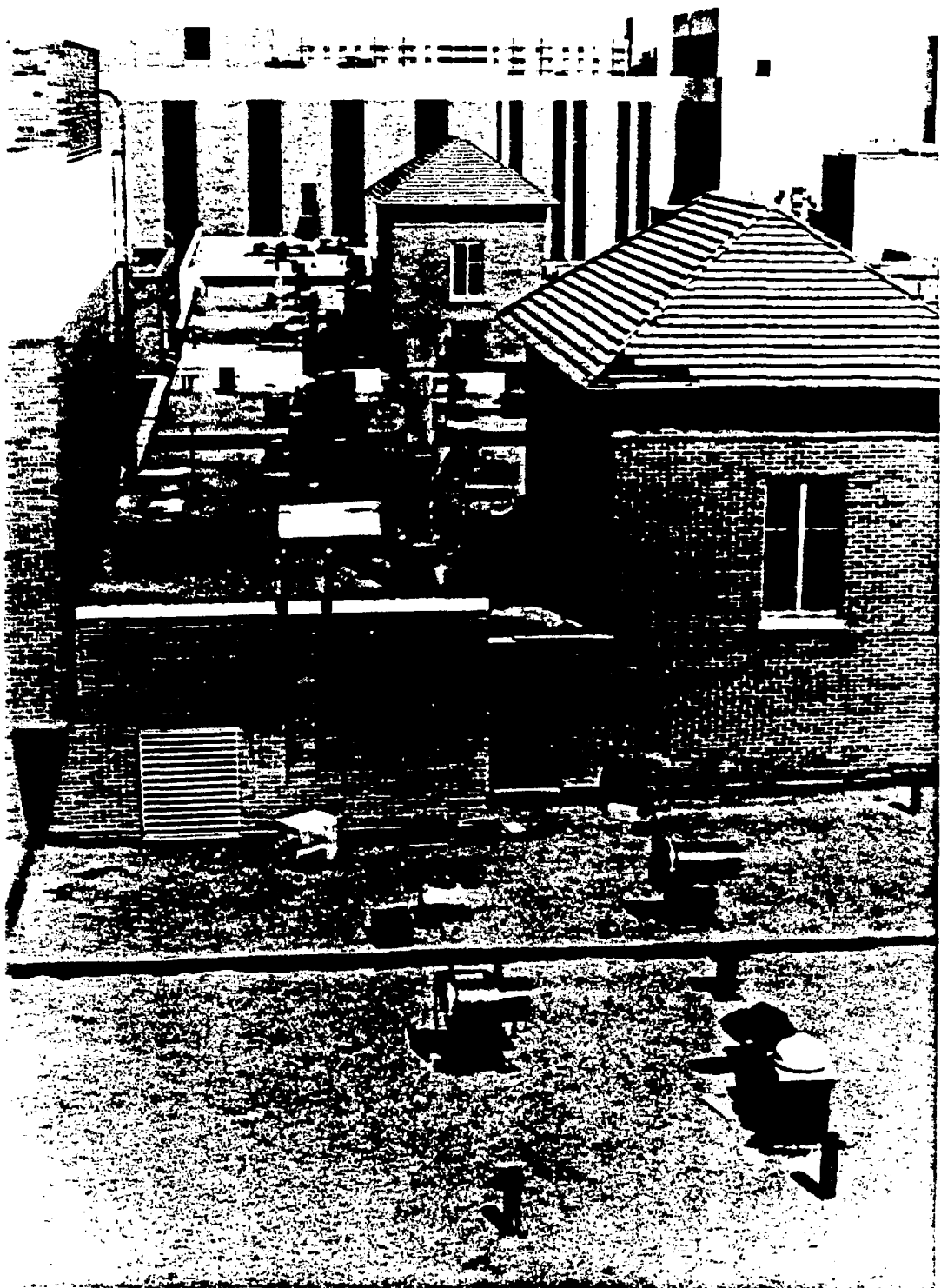
Figure 8 Effluent Release Points atop North Corridor
