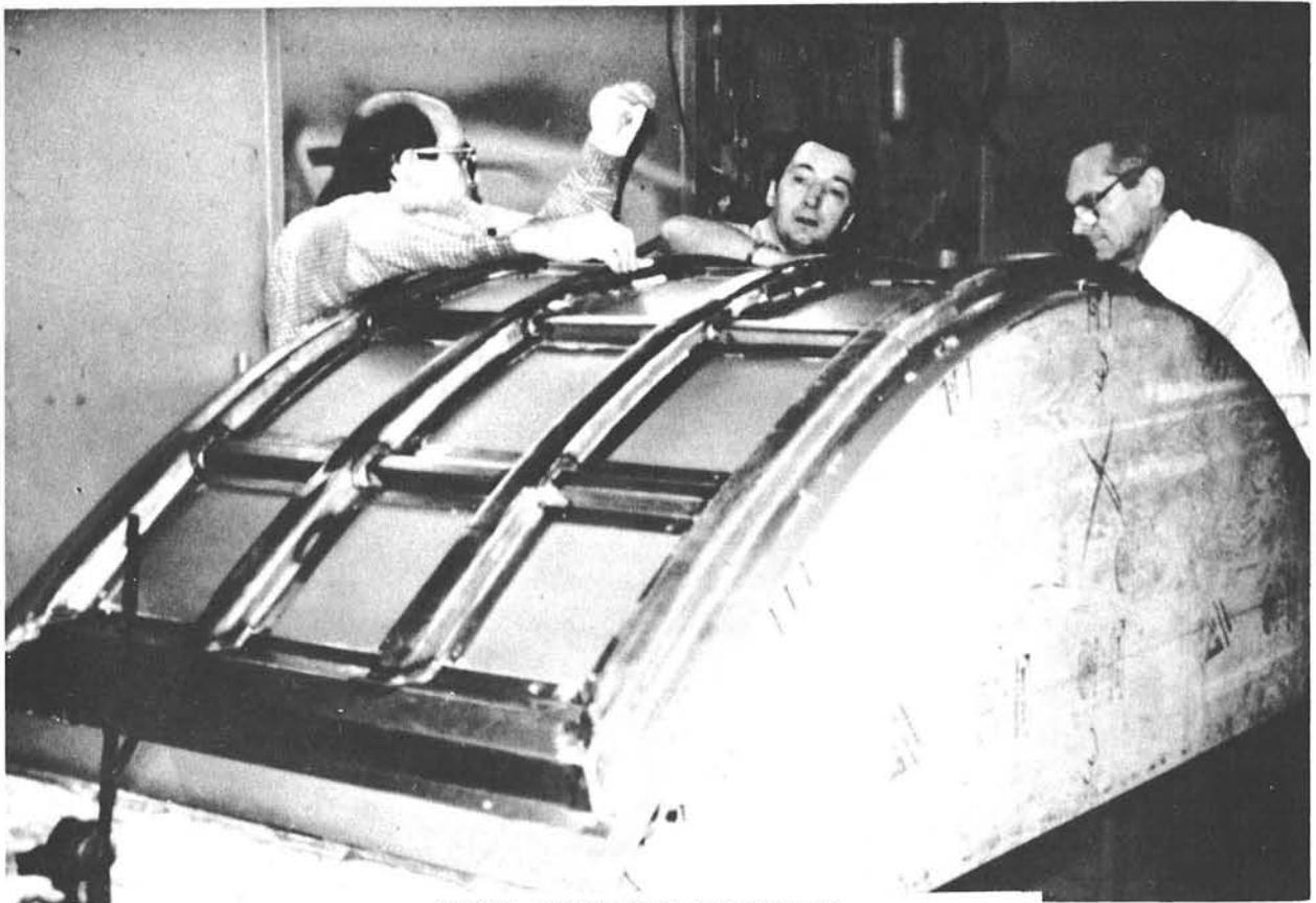
WOOD BONDING FIXTURE
