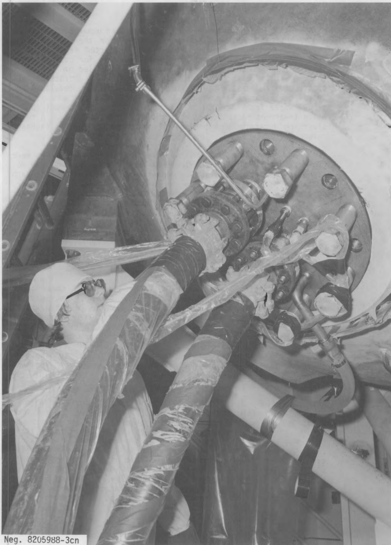
FIGURE 64. Manway Cover with Piping and Instrumentation Connections
