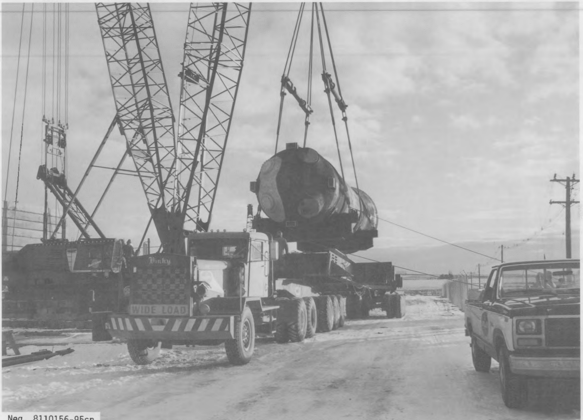
FIGURE 15. Lifting Generator Onto Trailer
