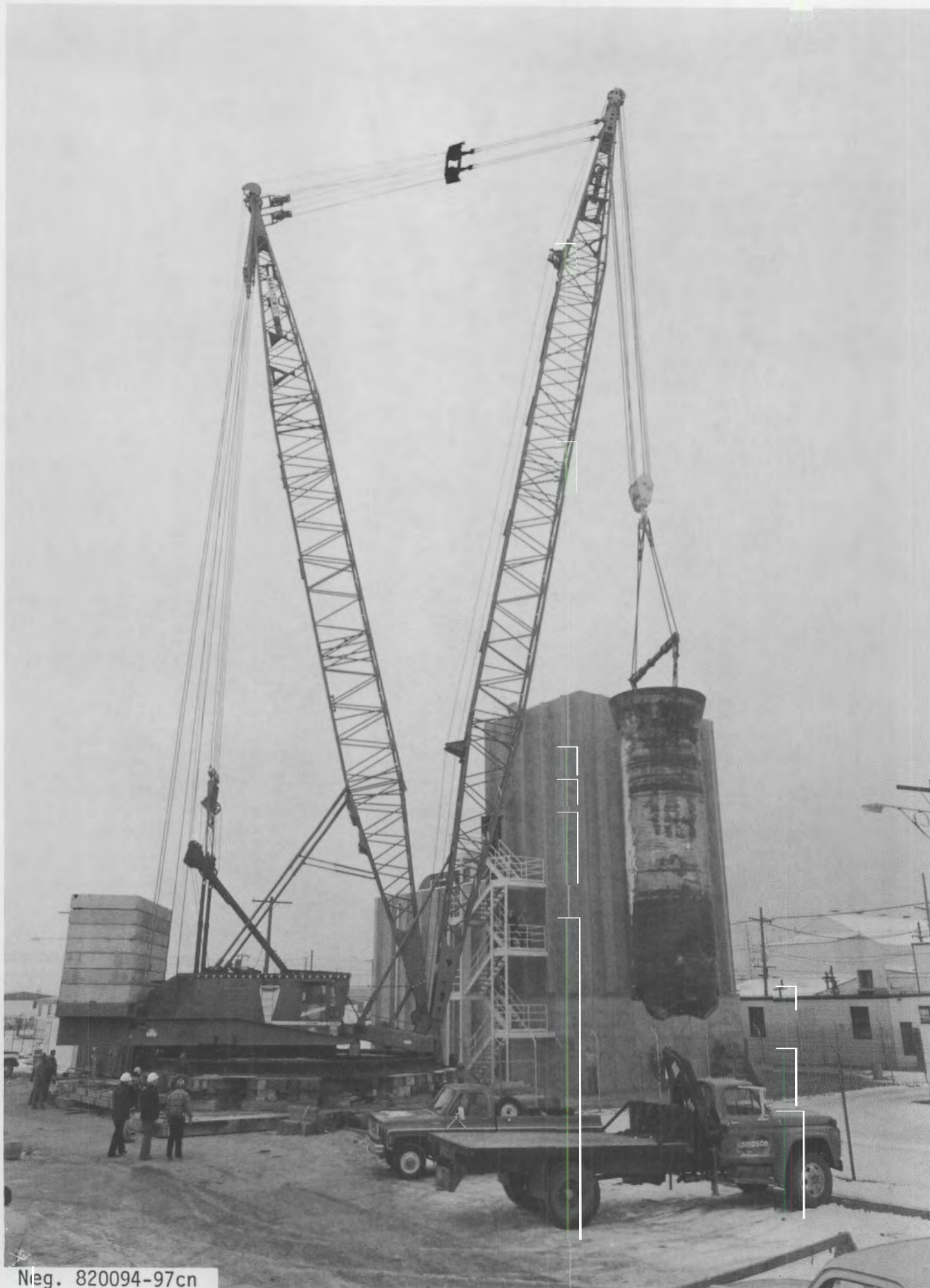
FIGURE 18. Lifting Generator Into SGEF
