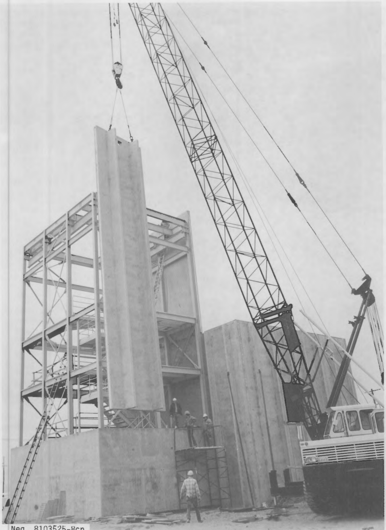
FIGURE 5. Placement of Tilt-Up Slabs
