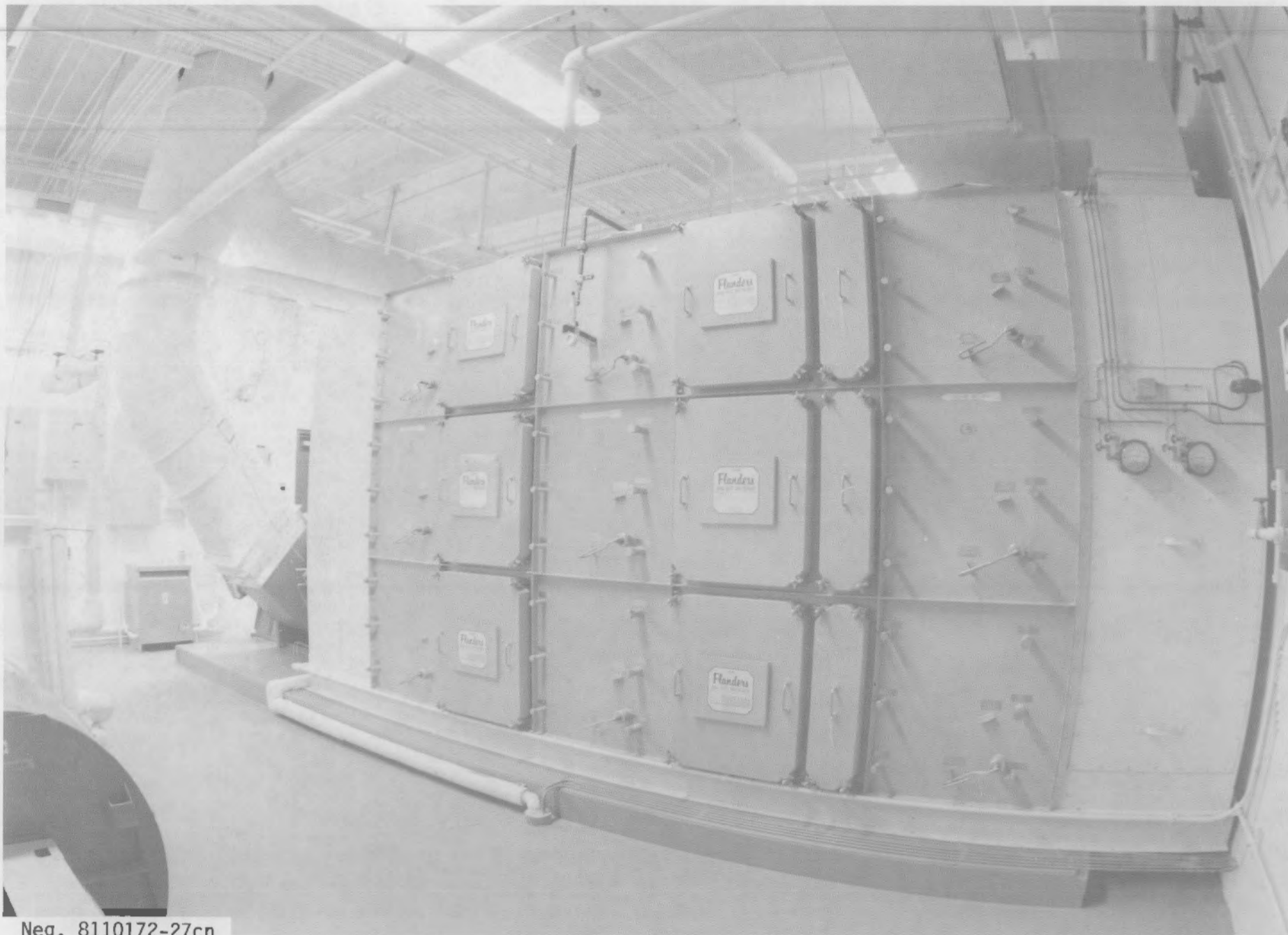
FIGURE 12. HEPA Filter Bank in Equipment Room
