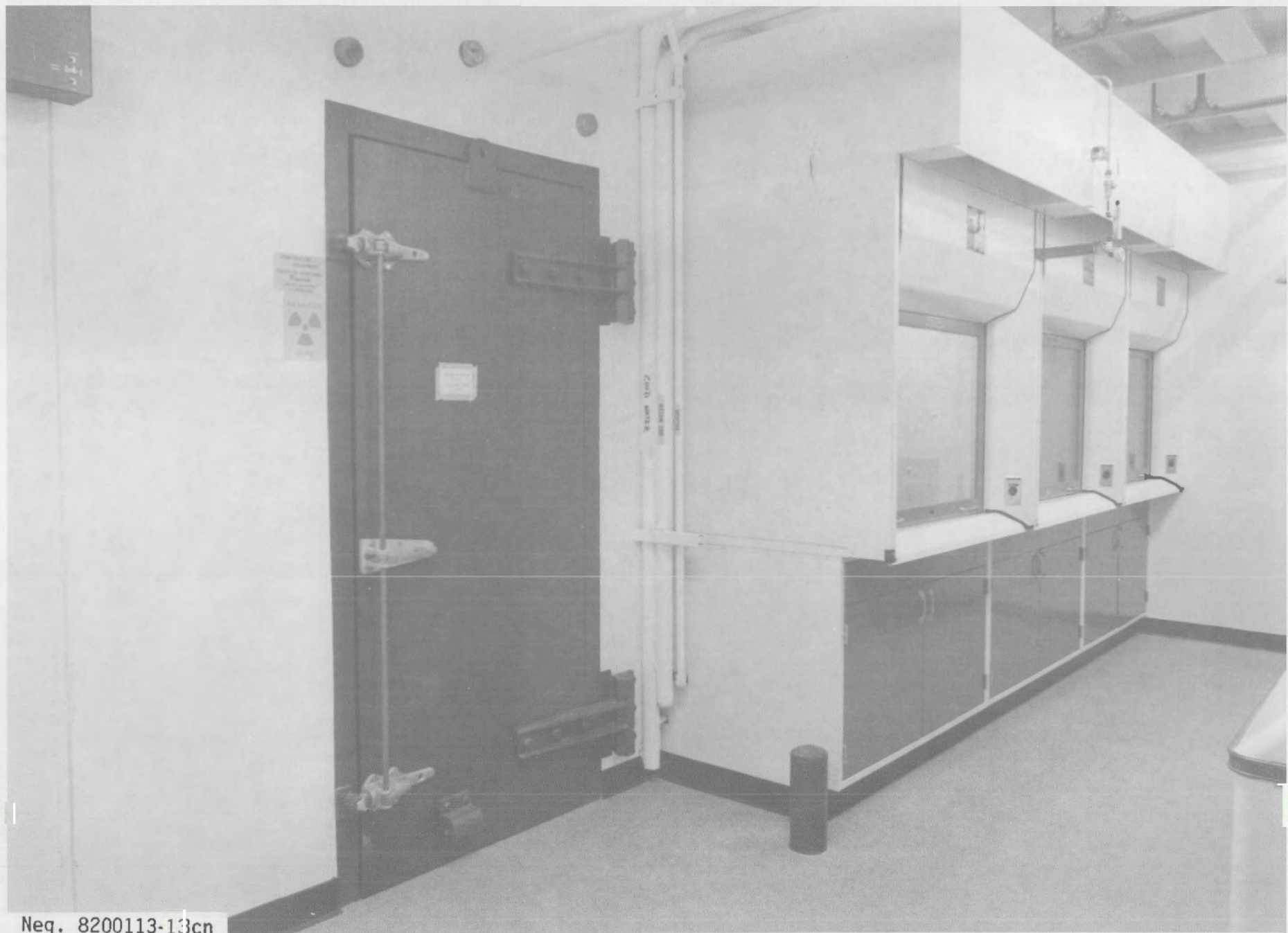
FIGURE 11. HEPA-Filtered Laboratory Hoods, Access Door to Tower
