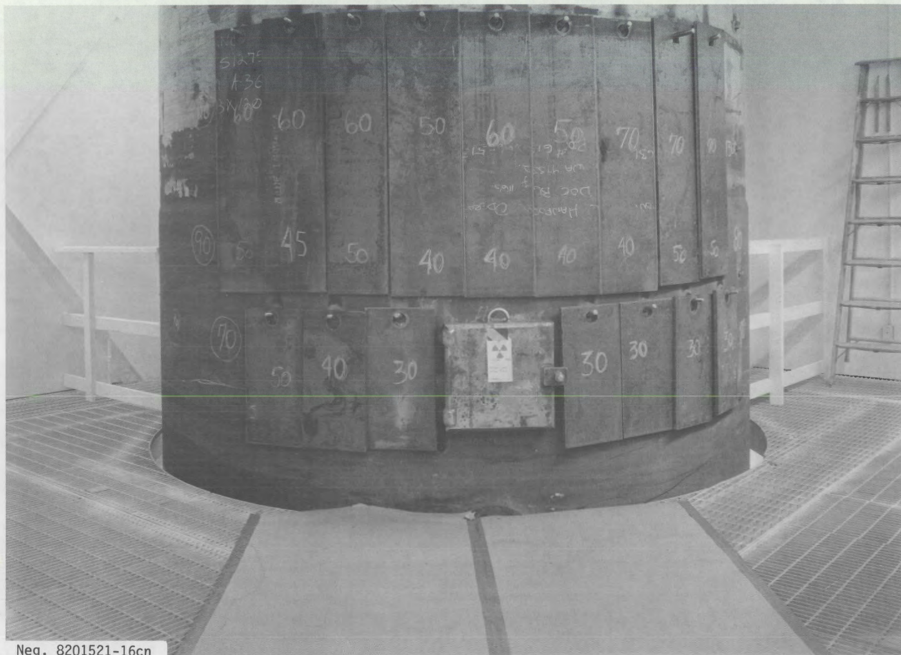
FIGURE 40. Shielding Arrangement in SGEF at Cut 1
