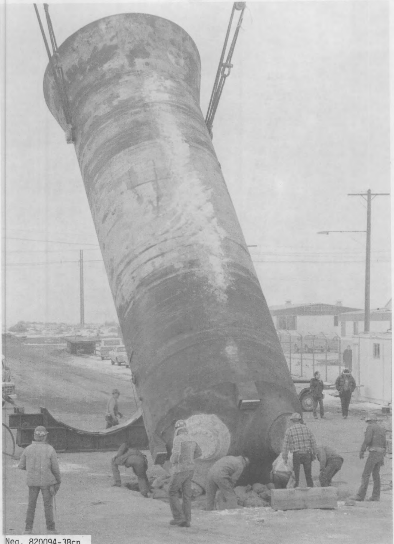
FIGURE 17. Sand Bag Pit for Upending Generator
