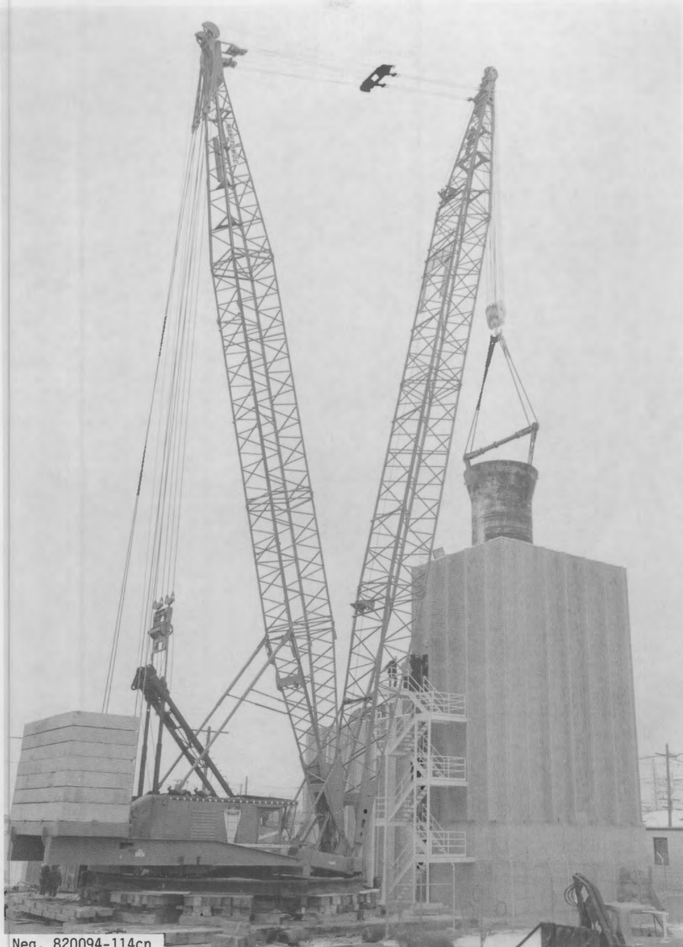
FIGURE 19. Lifting Generator Into SGEF
