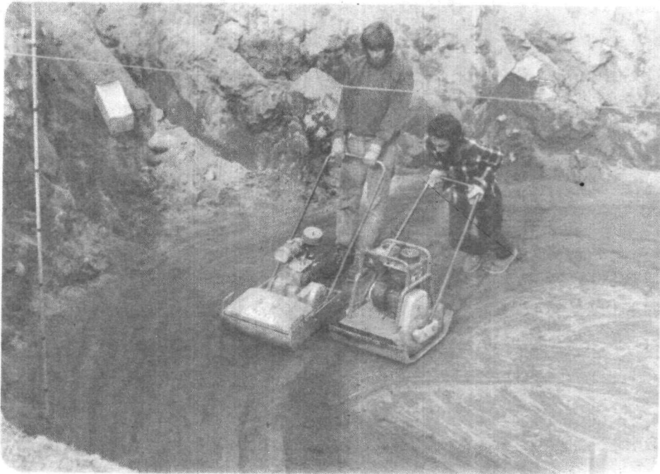
FIGURE D-2 COMPACTION
