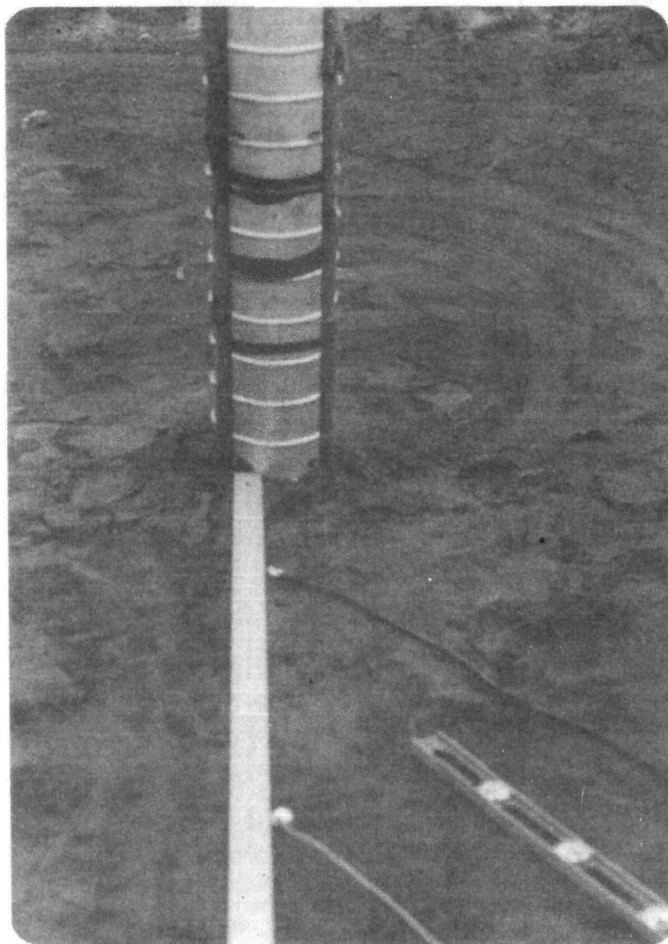
FIGURE D-7 INSTALLATION OF SENSORS AT EL. - 6.75 FT.
