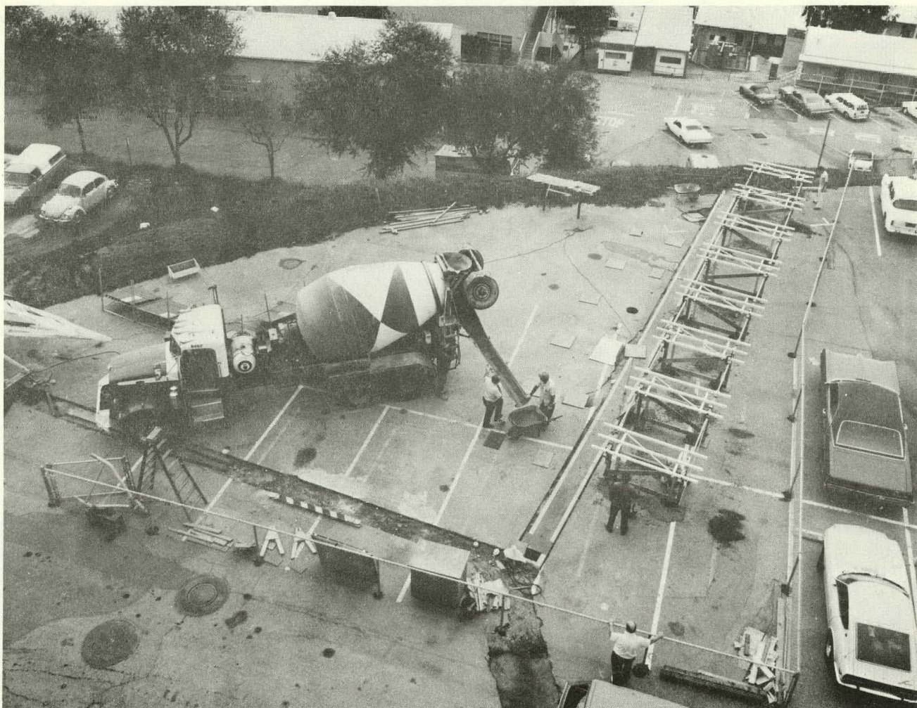
Fig. 5-9. Stands being installed at JPL Site
