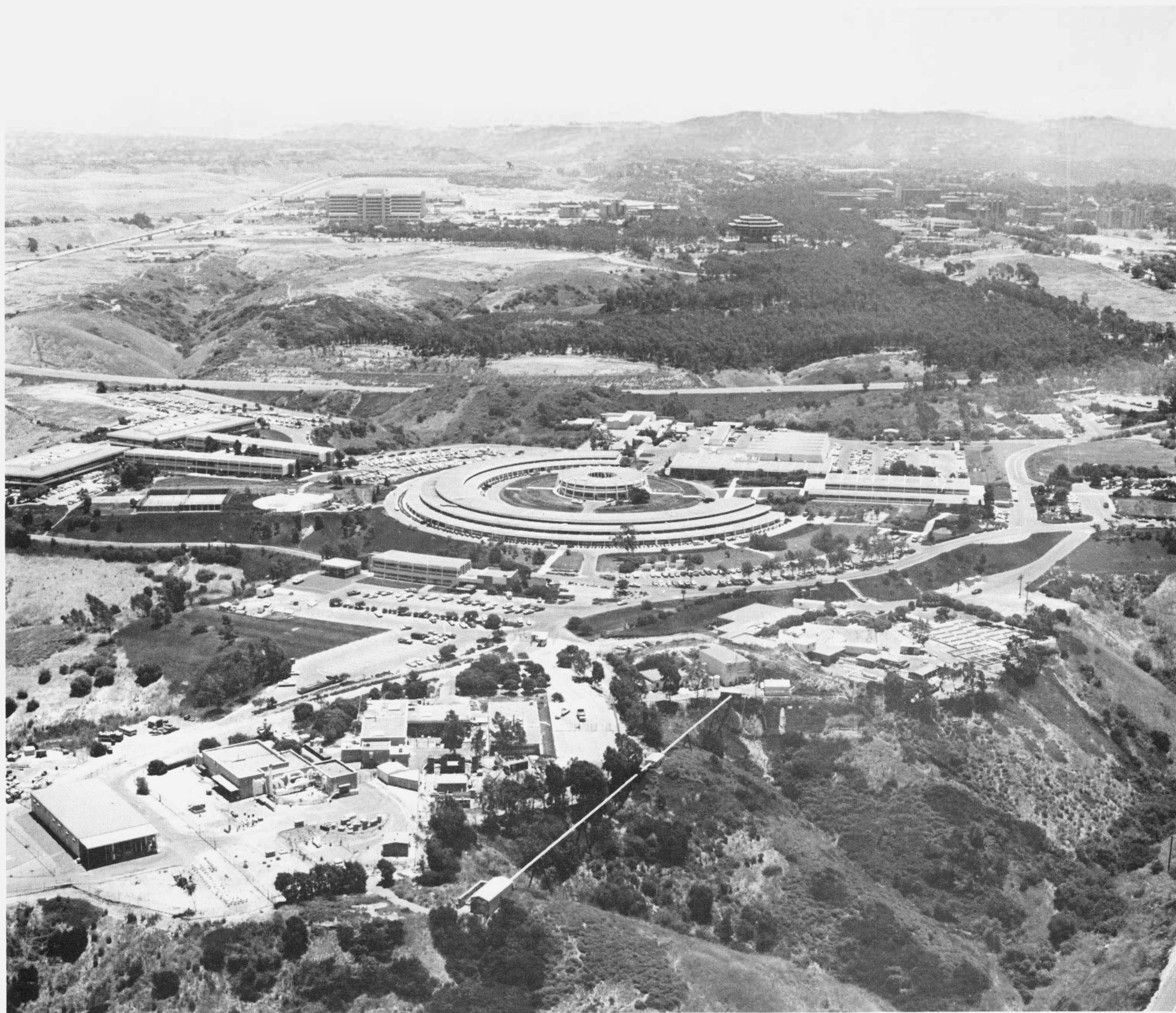
Figure 2. OBLIQUE PHOTOGRAPH OF MAIN GENERAL ATOMIC FACILITIES
