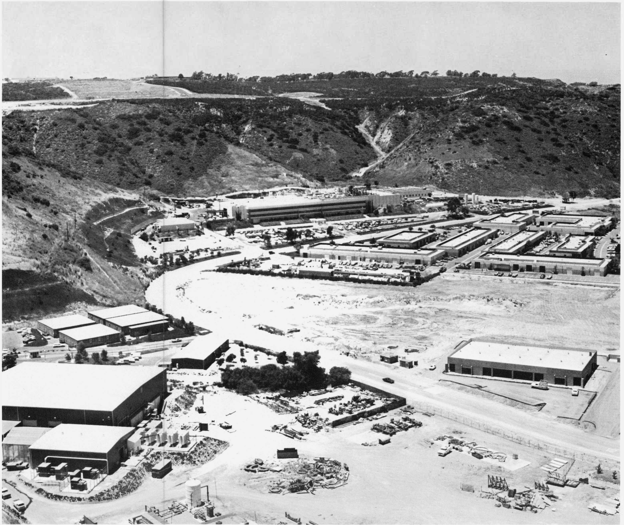
Figure 3. OBLIQUE PHOTOGRAPH OF GENERAL ATOMIC FACILITIES IN SORRENTO VALLEY
