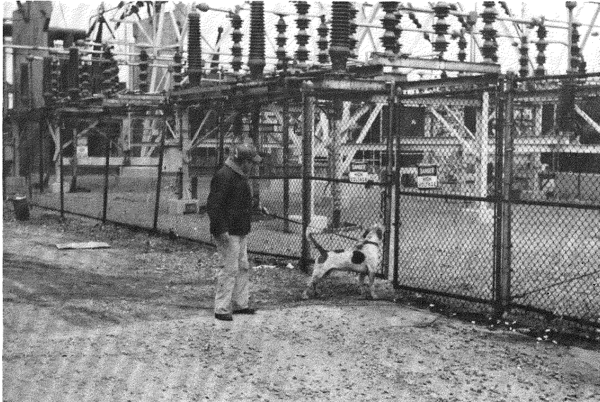
Figure 6.6. Woody Searching for Buried Leak
