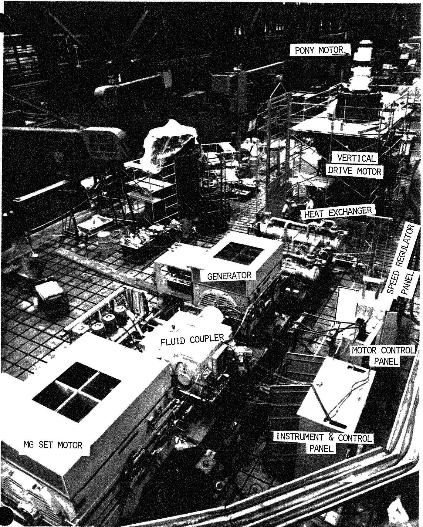
Figure 1.0.2.1 Sodium Pump Drive System Equipment Being Checked Out At GE Factory
