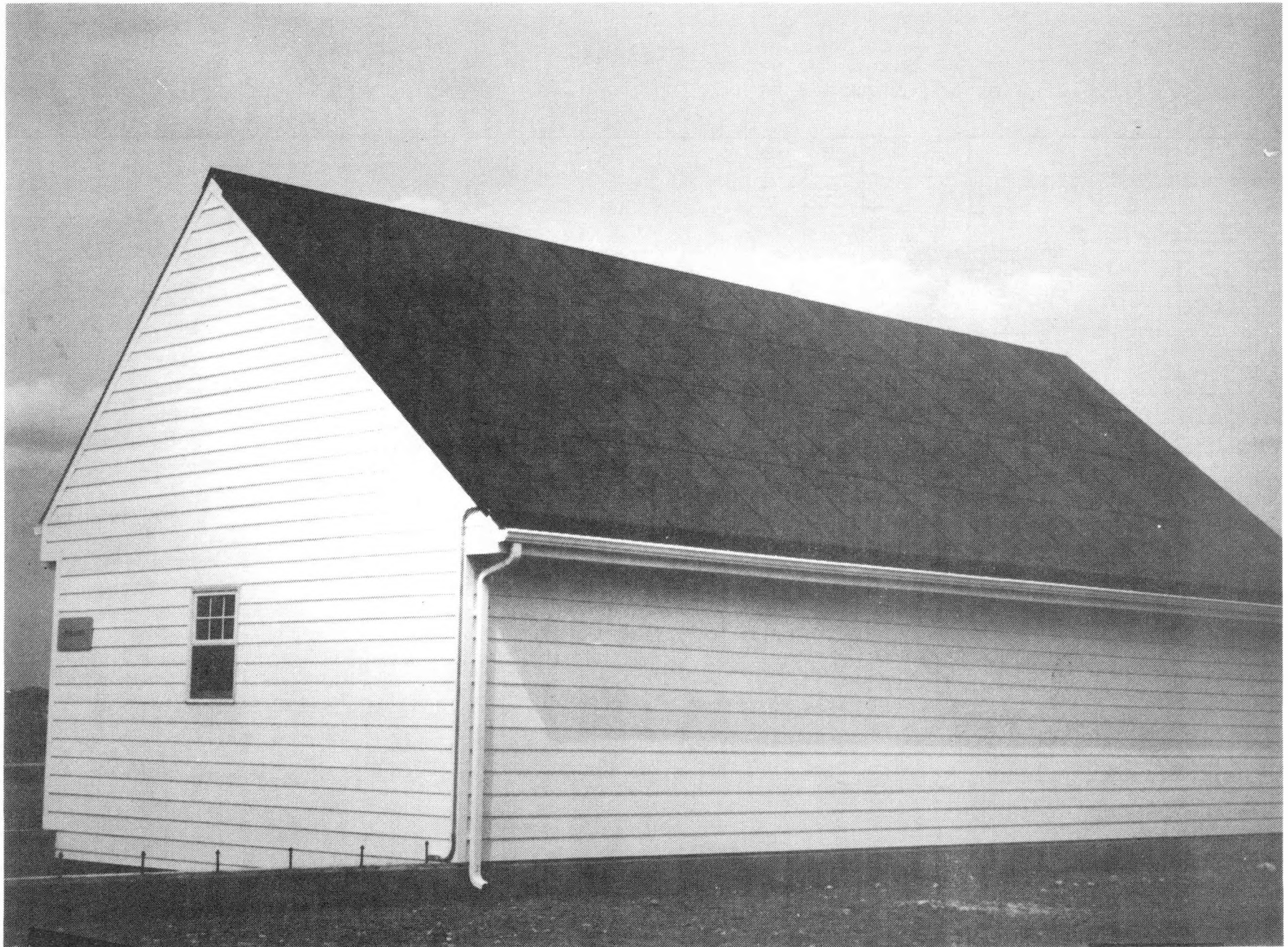
Figure 2.1.2-1 Photograph of the Prototype Residence at the Northeast Residential Experiment Station
