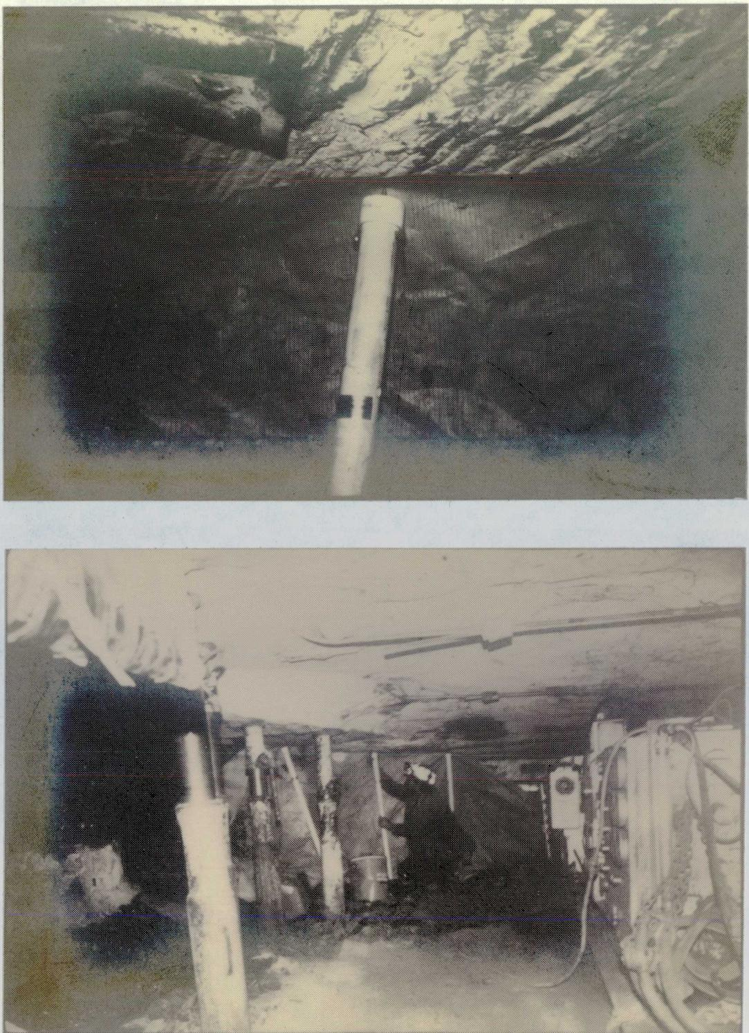
FIGURE 19. - Use of "Pogo Sticks" for wing curtain installation.
