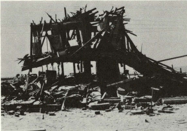
Unreinforced brick house after a nuclear explosion (1.7 psi peak overpressure)
