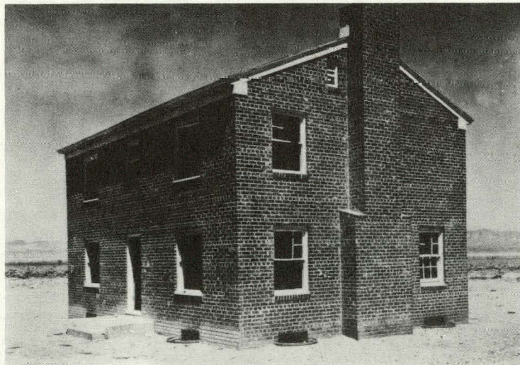
Unreinforced brick house after a nuclear explosion (5 psi peak overpressure)
