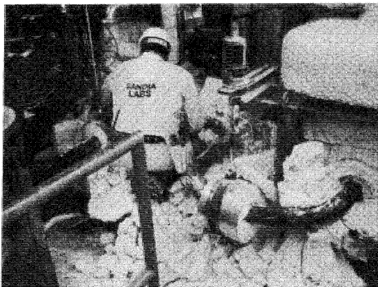
Figure 9. Repair of a burned out heat trace cable
