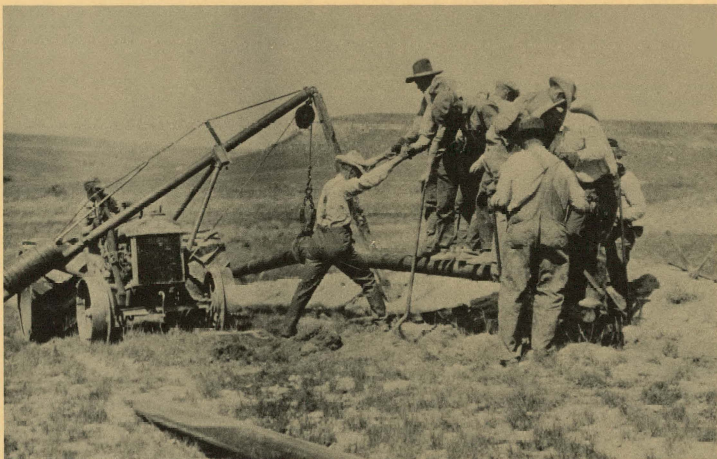
Early pipeliners lower pipe into a ditch near the Oklahoma panhandle in this 1938 photo. Note the counter-weighted rigging on the Fordson tractor used to assist the pipeliners.
