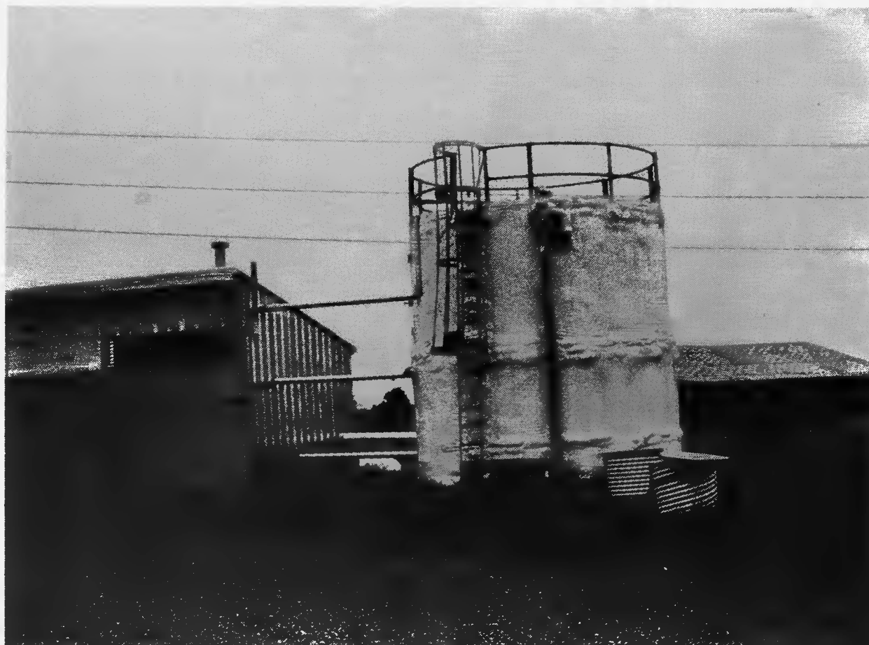
Figure 5. 21,000 Gallon Simple Complete-Mix Digester in Bedford, Virginia. Bumps showing through the bottom half of the tank are pipes carrying warm water to heat the digester. Adjacent building houses cogeneration equipment.
