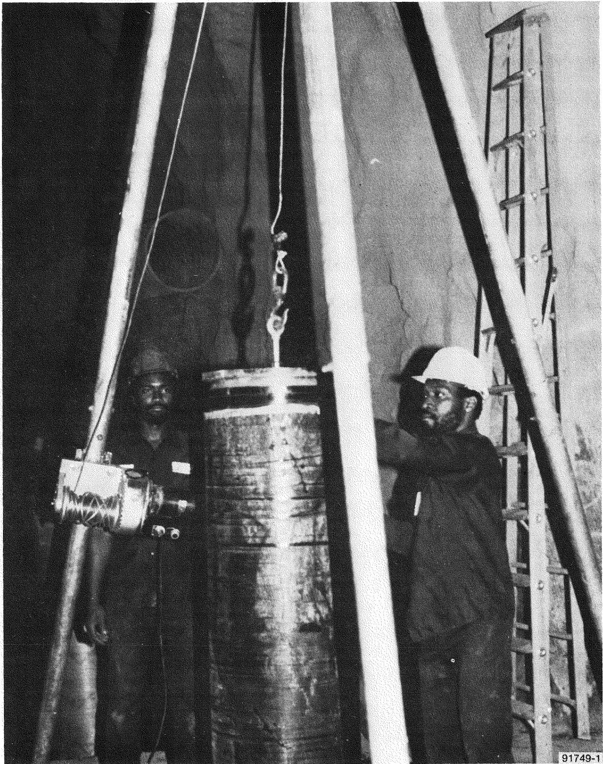
FIGURE 17. Retrieving Impression Packer from Full-Scale Heater Test #2 Main Heater Hole.
