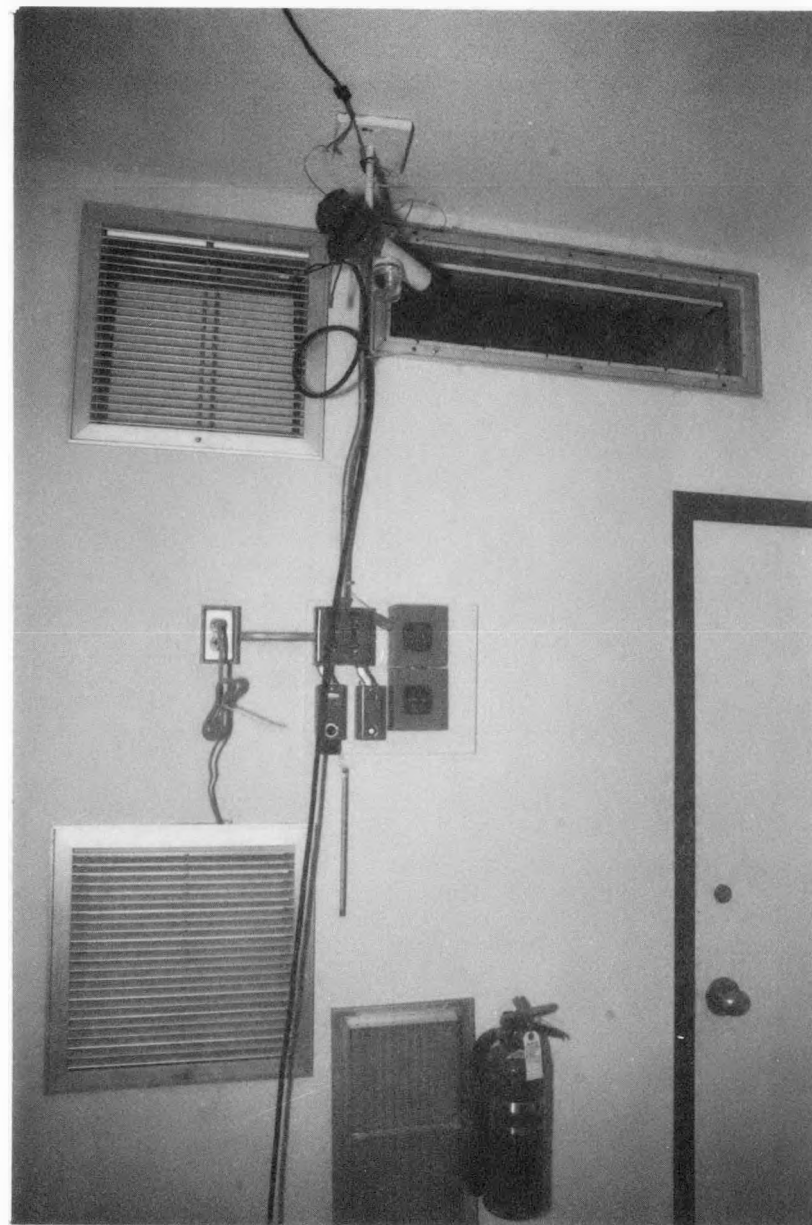
Figure 12. Controls and vents for attic solar collector system; open vent at top is for evaporative cooler
